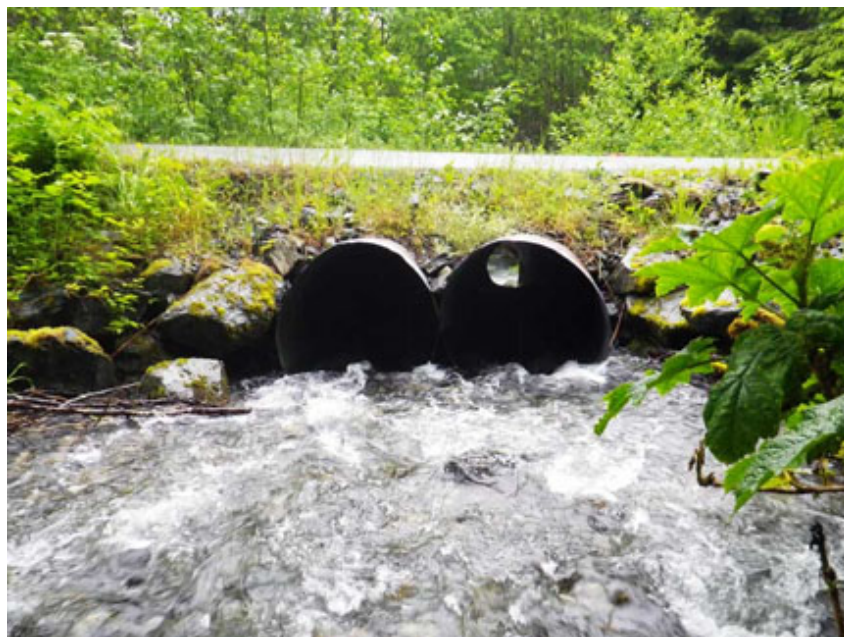
Figure 36.–Photograph of inlets from upstream.
