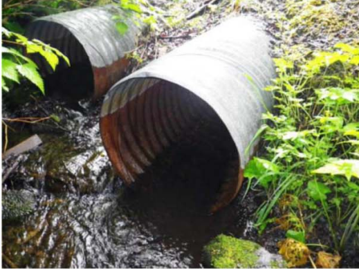
Projecting Culvert
