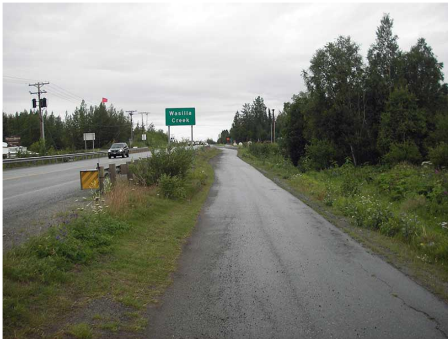
Figure 32.–Photograph of road surface.
