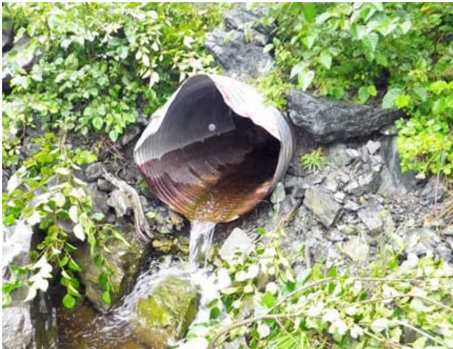
Figure 34.–Photograph of outlet from downstream, showing outfall type and condition.
