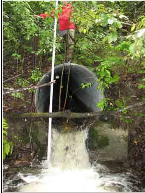
Figure 13c.–Projecting culvert with an outfall type: free-fall into pool.
