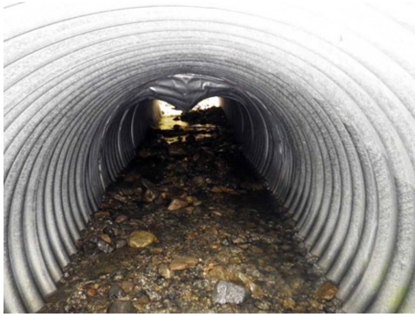
Figure 37.–Photograph of the inside of a culvert.
