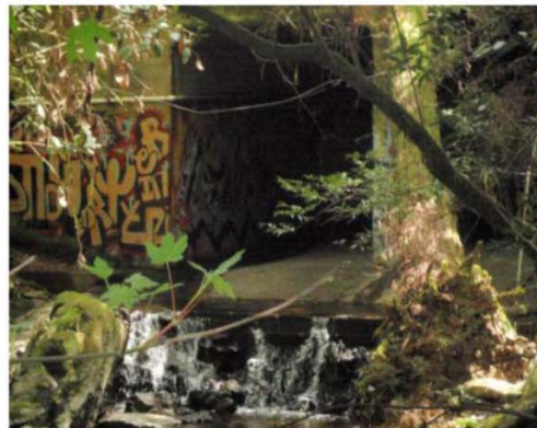
Concrete Apron Culvert
