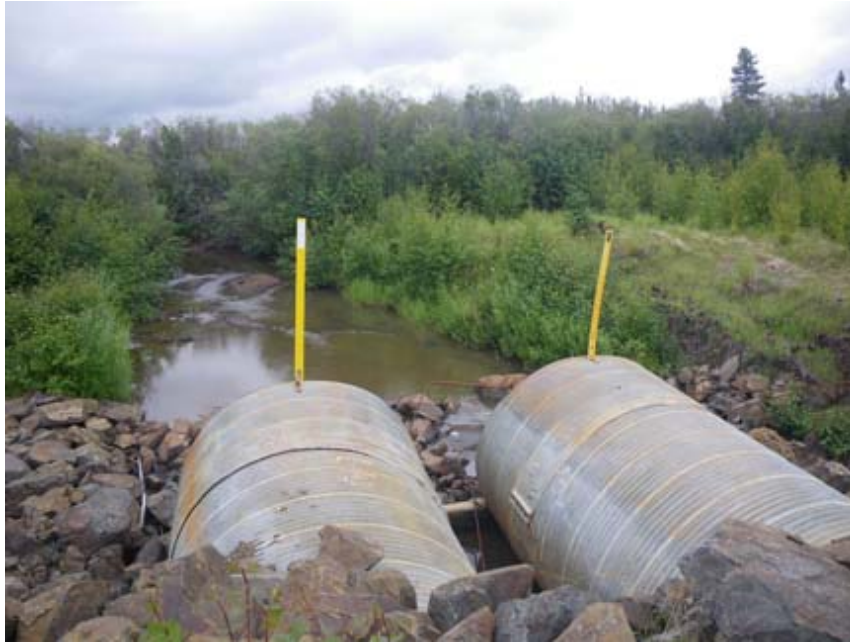
Figure 33.–Photograph of inverts from road looking upstream.
