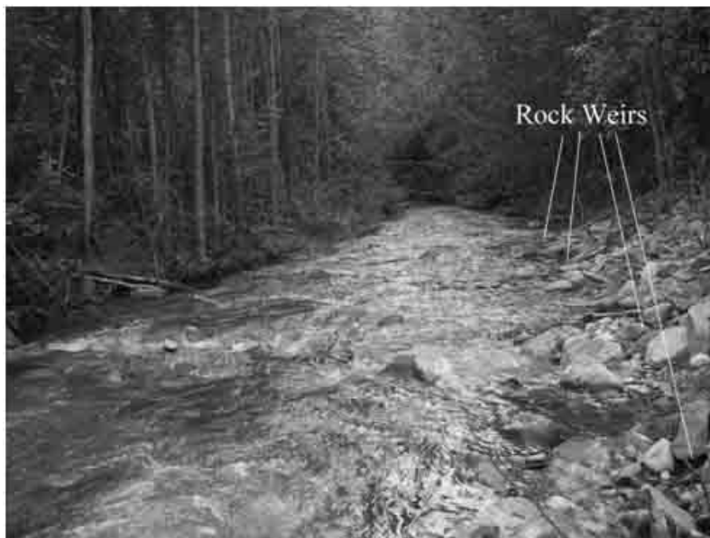
Figure 26.–Photograph showing constructed rock weirs downstream of culvert.
