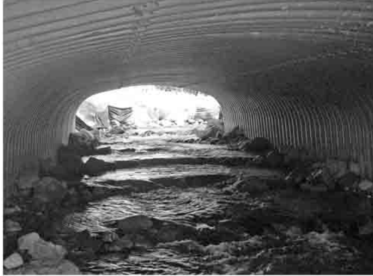
Figure 25c.–Constructed step pools running through an embedded culvert.
