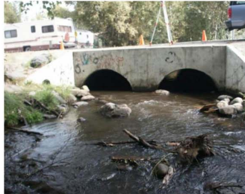
Wing Wall Culvert
