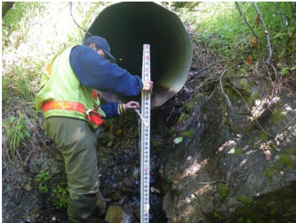
Figure 35.–Photograph of outlet with a measuring rod for reference.
