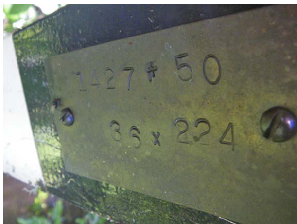
Figure 29.—Department of Transportation placard on culvert marker.
