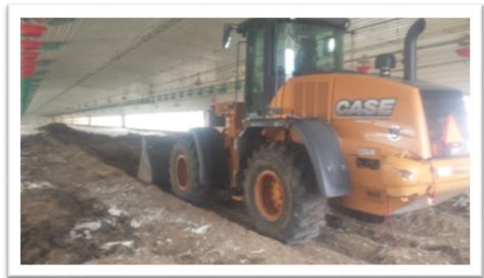
Pay loader used for clearing the base (photo by Josh Payne)
