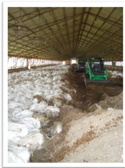
Clearing the base (photo by Gary Flory)
