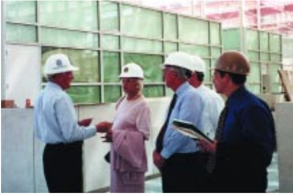
Justice O'Connor, John O'Connor, Judge McNamee and Judge Broomfield tour the court building during construction in August.
