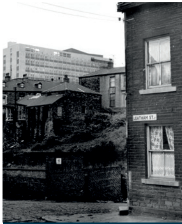
The Victorian streets shortly before demolition, with the University's Richmond building in the background. Copyright Special Collections, University of Bradford UNI X325/5/1/9
