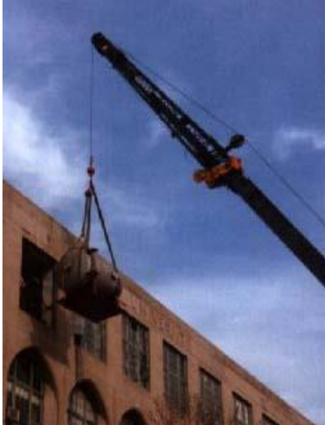
Vacuum tank being lifted into the CAS building
