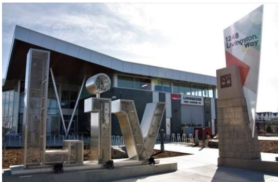
New Livingston Response Station in N.E Calgary
