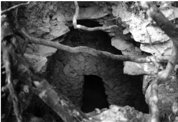
Figure 9. Photograph of the interior of Structure 1, showing Chamber 1 and the doorway (1 m in height) into Chamber 2. Photograph by Villamil.
