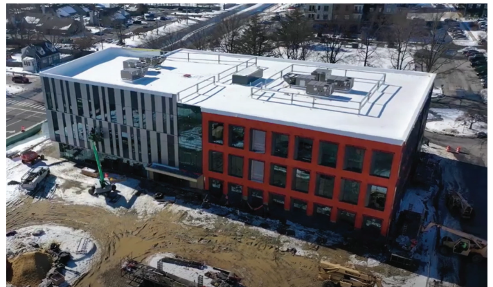
Courtesy of Marlette/BPGS Construction, Marlette's new Delaware office.
