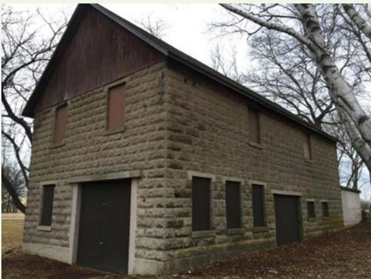
Above: Park shelter and stone barn.
