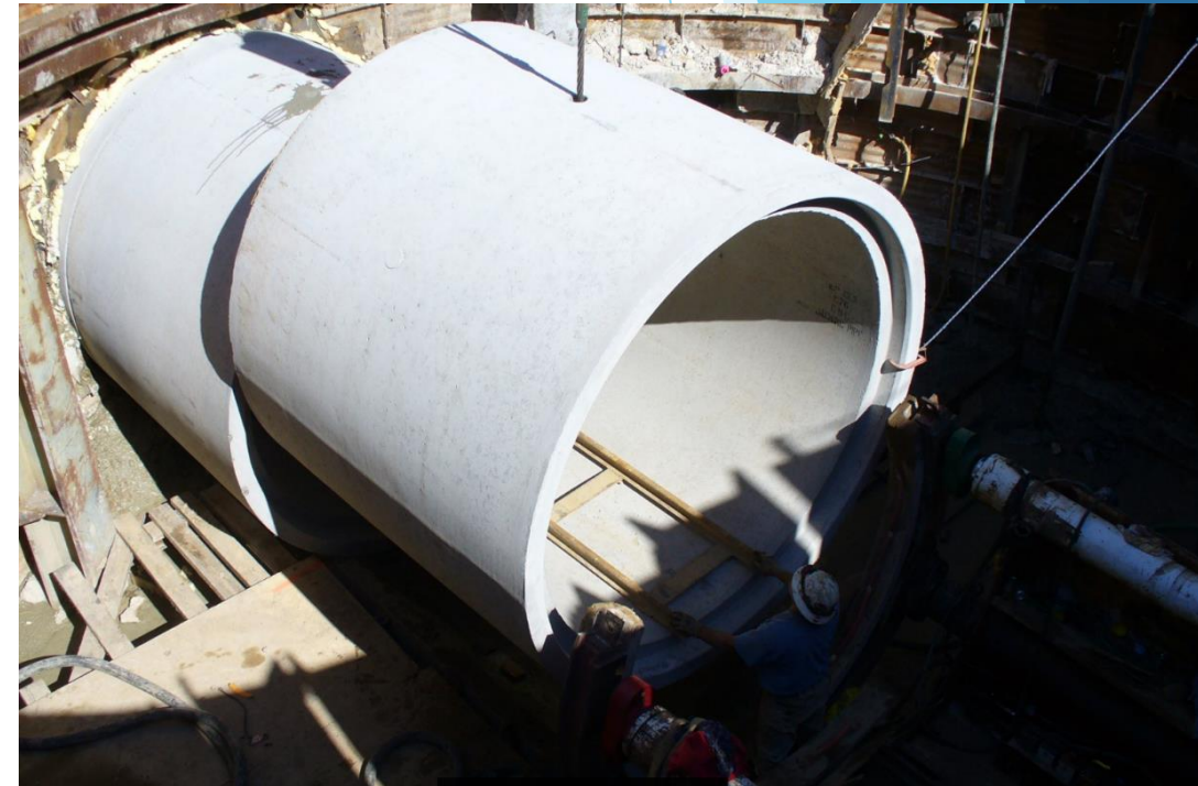
96" pipe tunneling on University Ave, Madison, WI (2013)
