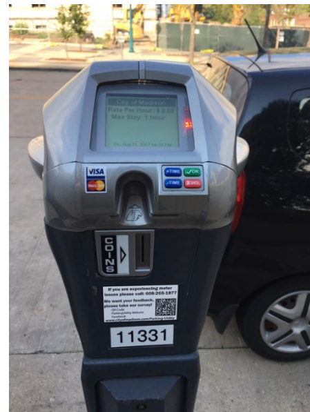
Figure 27 Smart Meter Conversion
