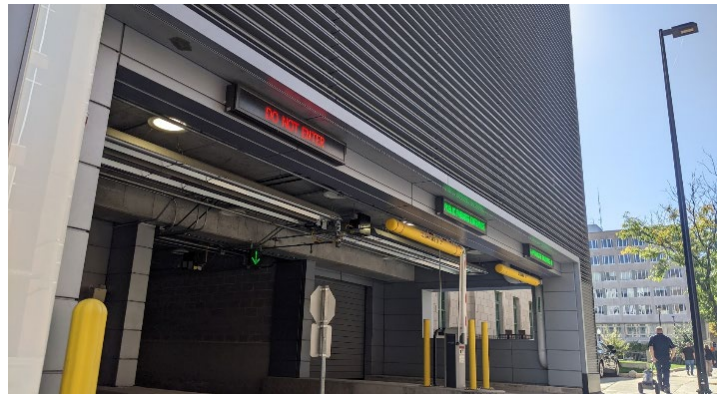
Figure 26 Wilson Street Garage Repairs
