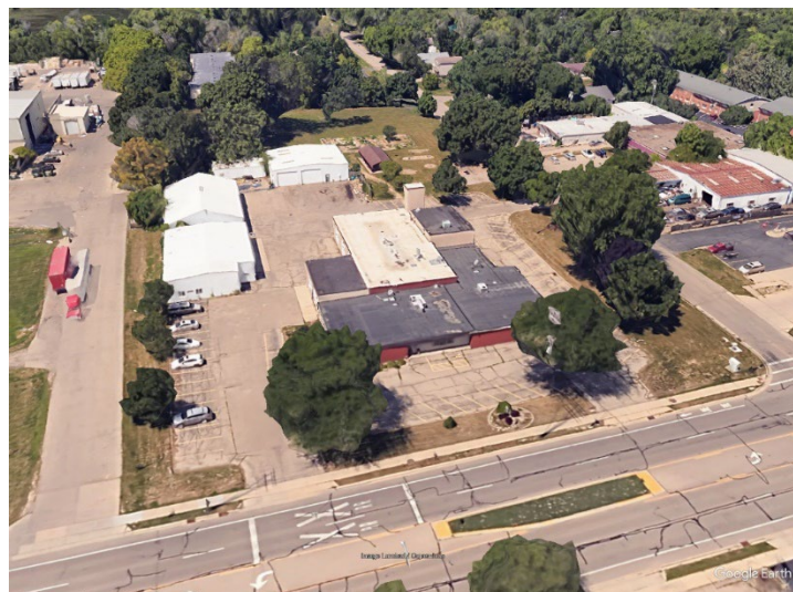
Figure 31 PEO Relocation to the Former Town of Madison Bldg
