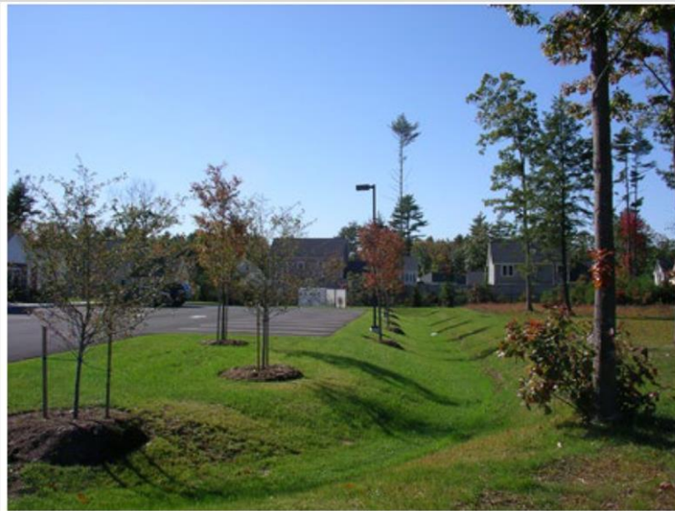
Grassed bioswale in New Hampshire.
