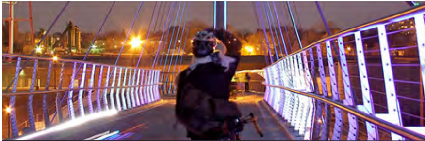
Hiawatha Bridge on the Midtown Greenway SOURCE: Tony Webster on Flickr
