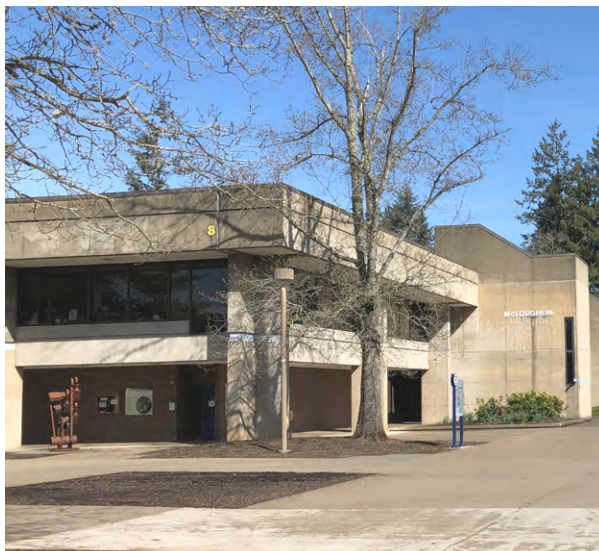
Existing view of McLoughlin Hall ground floor
