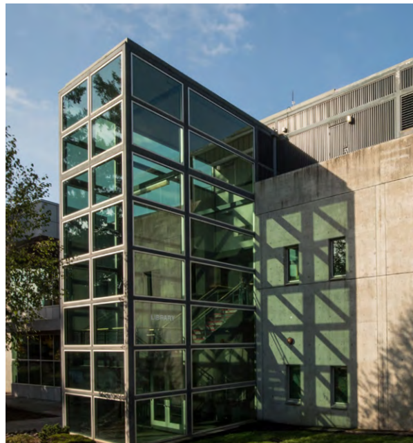
Example of a stair tower converted from concrete to glass.
