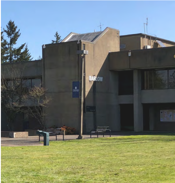
Existing Barlow Façade
