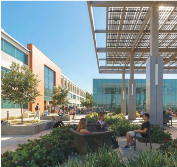
Solar arrays can be used as canopies above outdoor seating, providing electrical generation and multi-season outdoor space.
