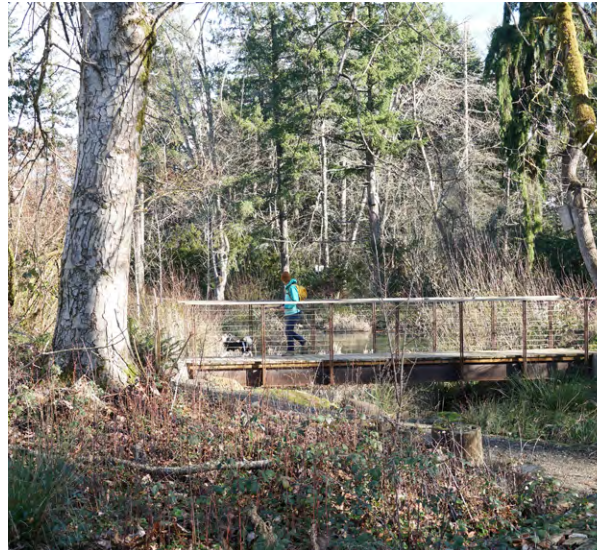
Bridge Crossing at Newell Creek
