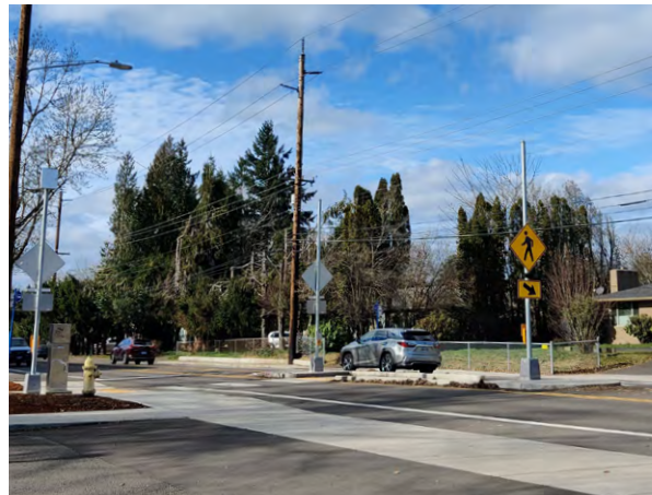
New pedestrian-activated crosswalk on SE Harmony Road
