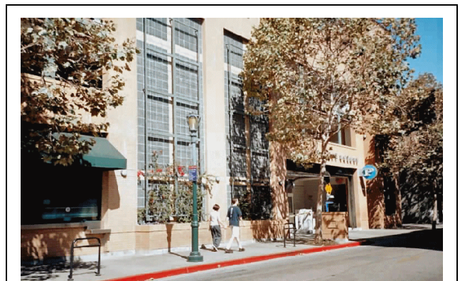
Figure 41. This parking garage includes street front retail space and landscaped trellises to mitigate visual impacts on the streetscape
