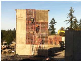
Construction progress on the Sammamish Community and Aquatic Center
