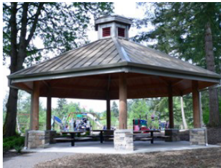
Shelter at Ebright Creek Park
