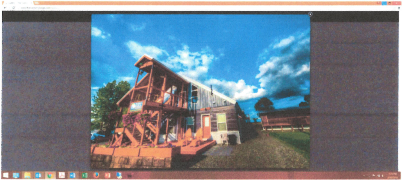
Original Lodge Liquor License 2 nd Floor of this Building Old Admin
