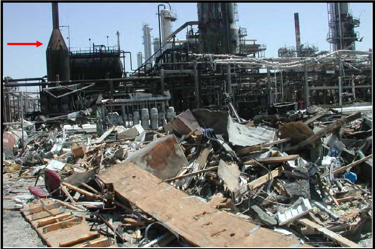
Figure 13. Destroyed trailers west of the blowdown drum (red arrow in upper left of the figure)
