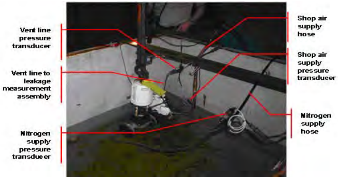
Figure S- 7. PCV-5002 shop testing
