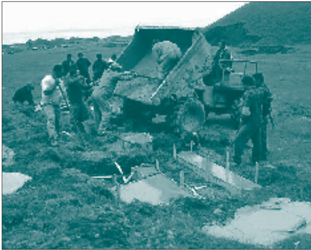
ISLANDERS HELPING TO BUILD INFRASOUND STATION IS49
