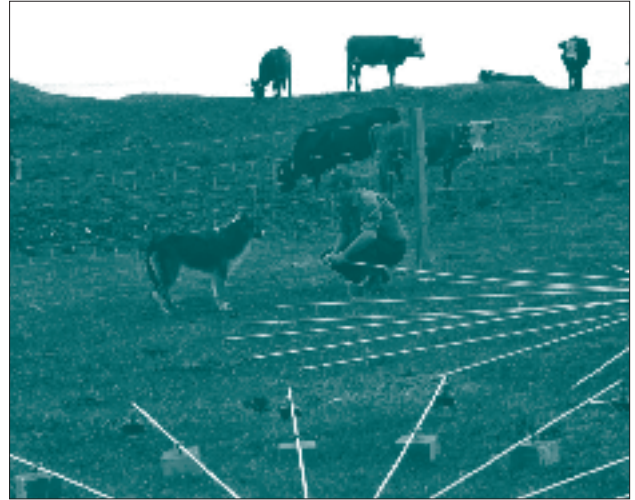
PTS STAFF INSTALLING PIPE ARRAY
