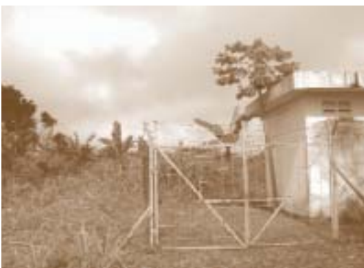
RELIMINARY SITE SURVEY OF A RADIONUCLIDE STATION IN EDEA (CAMEROON), AUGUST 2002.
