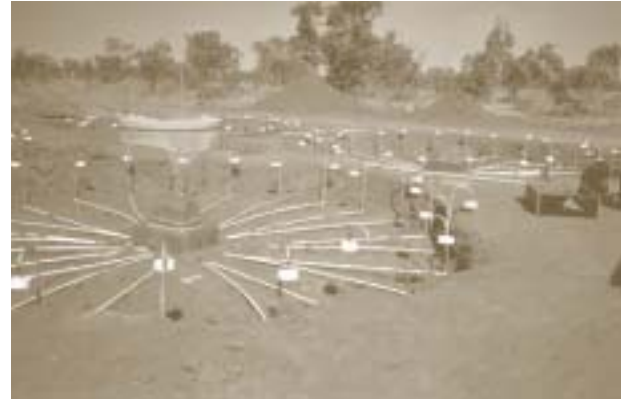
CONSTRUCTION OF WIND-NOISE-REDUCING PIPE ARRAYS AT INFRASOUND STATION IS07 WARRAMUNGA (AUSTRALIA)
