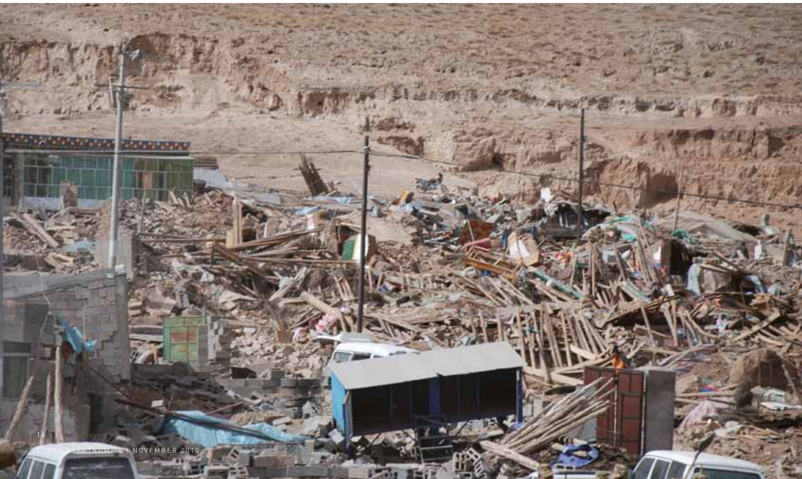
A 6.9 magnitude earthquake on 14 April 2010 caused devastation in Yushu county in western China's Qinghai province.
