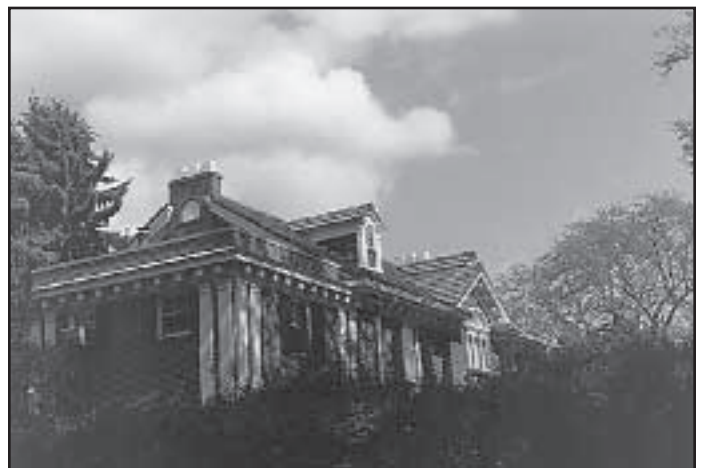
Highly textured roof materials are a character defining feature of the district.
