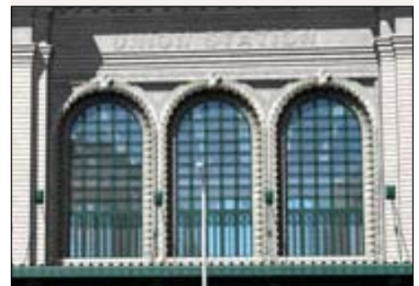
The 3 main windows along the eastern facade of the Station
