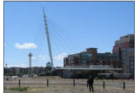
The Millennium Bridge over the CML
