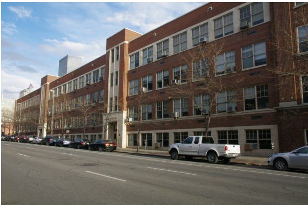
11. The historic structure conveys high quality design and materials, including brick and terra cotta. The building also displays a high level of façade articulation and visual interest, such as projecting bay towers and horizontal window expanses.
