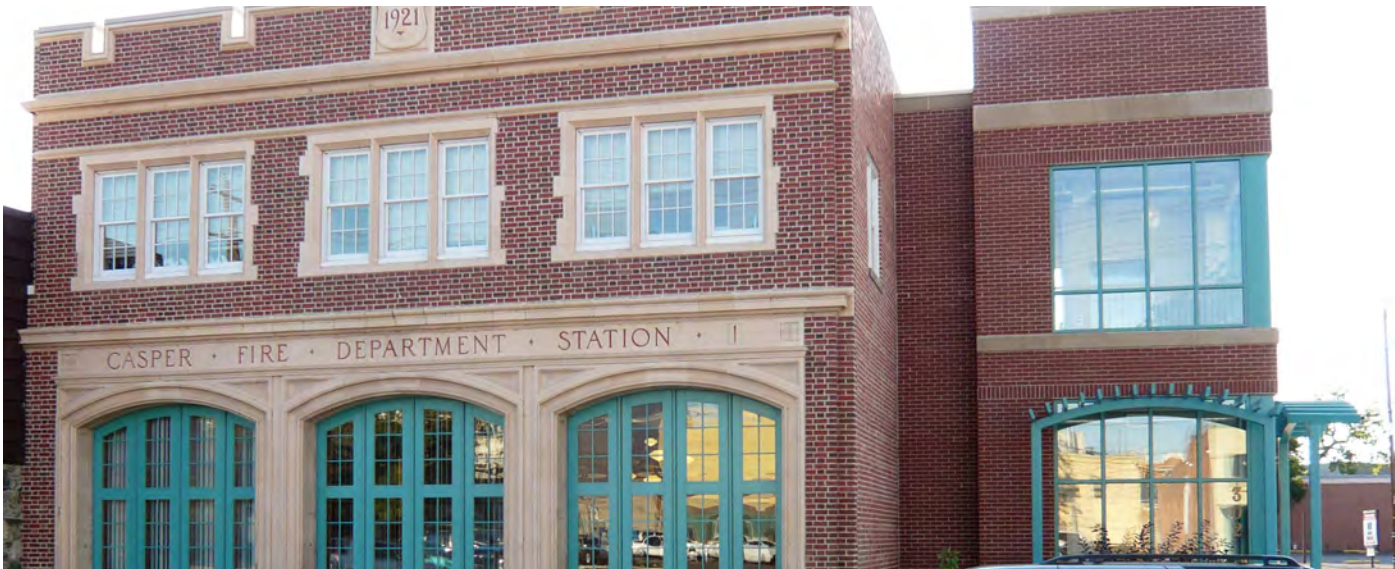
A contemporary addition, on the right, to an historic Fire Station in Casper. The addition features a change in wall plane and similar window and door proportions that complement the original windows and doors. The addition has simplified ornamentation.
