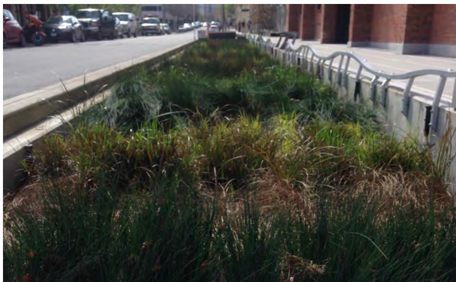
Water quality planters filter pollutants and debris from stormwater runoff, providing a valuable service to the city. To maintain proper functioning, these devices need regular maintenance, especially after a storm event.
