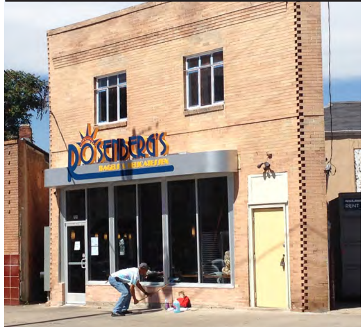
AFTER - E 26TH AVE FACADE
