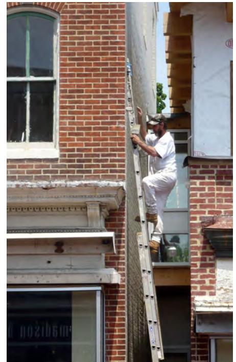
Rehabilitation work underway on an historic building.
