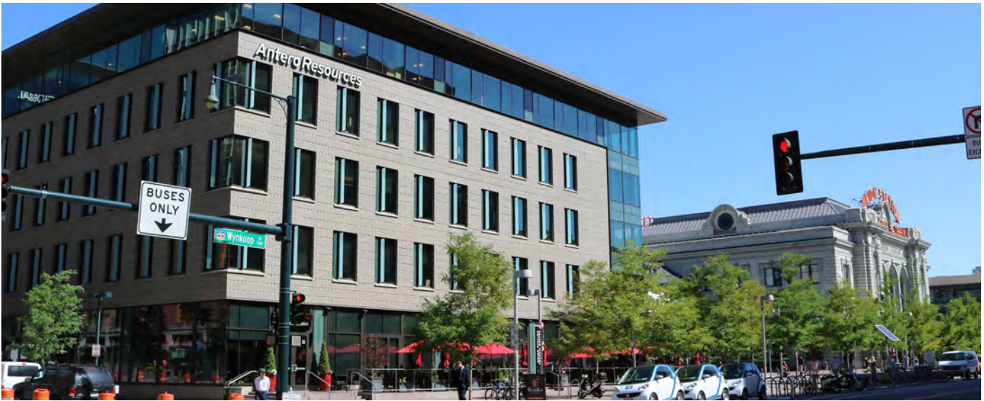
A fully articulated facade on infill construction with a defined storefront base, punched upper floor windows with sills, horizontal orientation, and a differentiated upper floor above three-stories.
