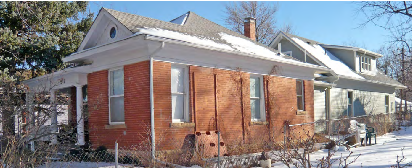
A rear addition to a residential structure with a compatible roof form and a differentiation in material.
