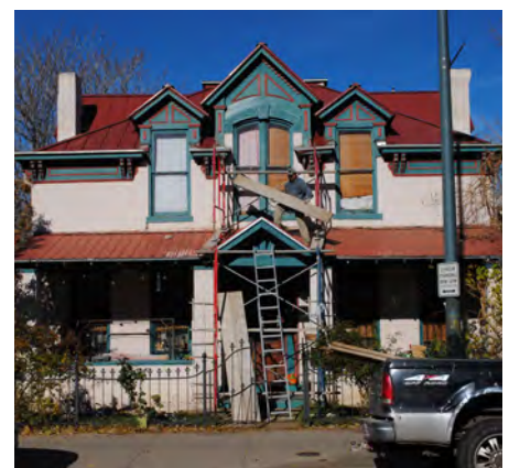
Scaffolding for repair work on a building.
