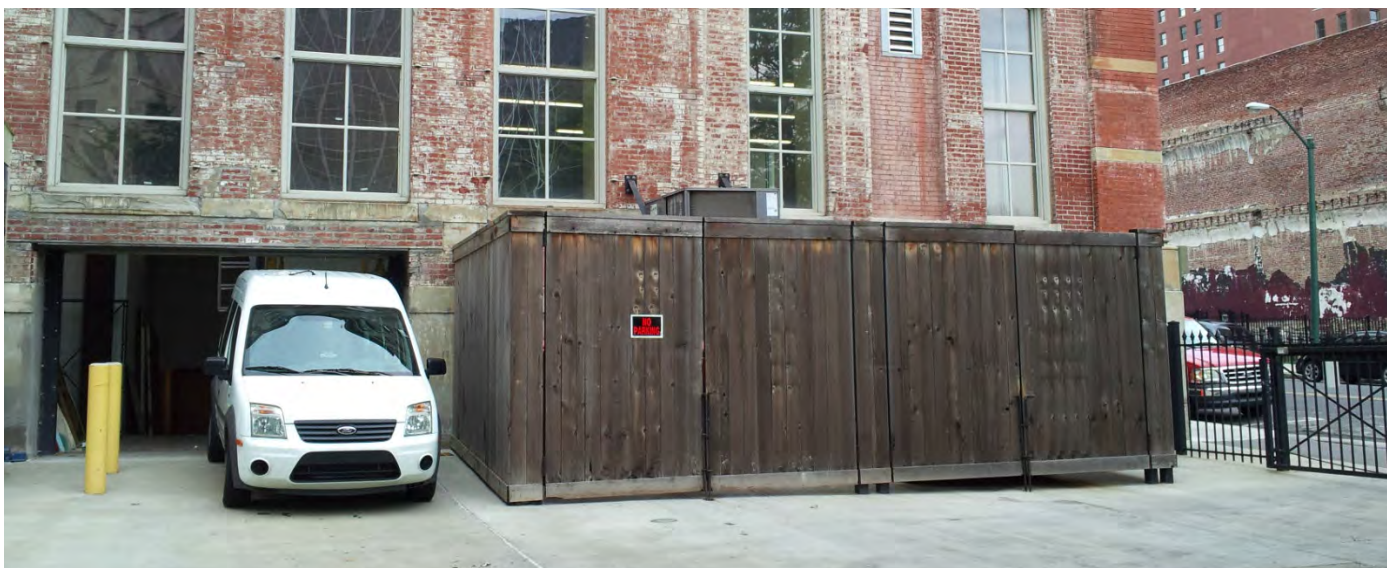
Screen utilities and service areas to maintain a high-quality pedestrian experience.
