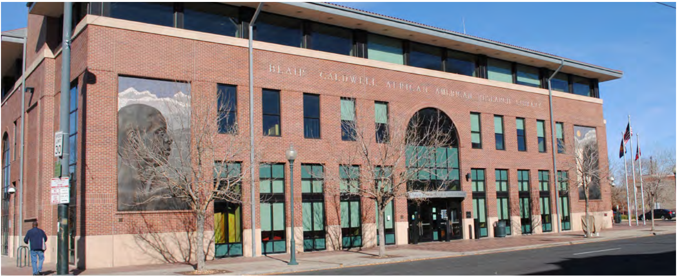
The Blair-Caldwell African American Research Library is an example of post-1964 construction. It has a clearly defined primary entrance covered with a canopy, red brick construction, punched windows, and public art along the facade providing visual interest and a cultural reference.
