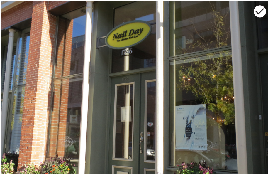
1. This signage was installed to limit impacts to character defining features of the building, such as the cast iron columns.
