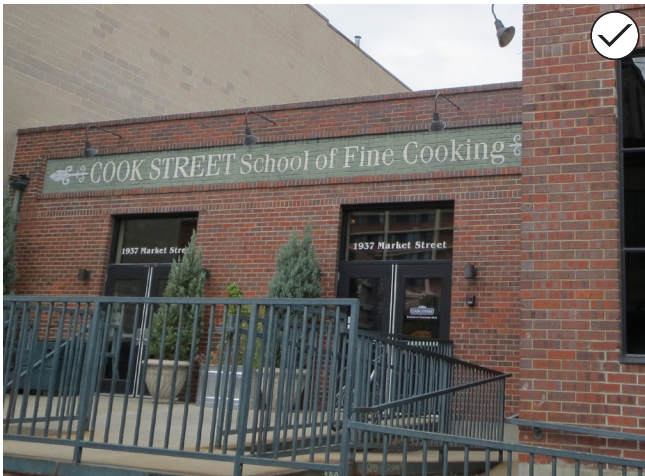
21. When using an existing sign band, provide space between the sign and the sign band edge. Keep sign flush with painted or pin mounted letters.
