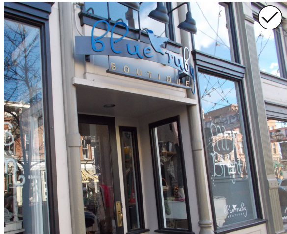
22. A slightly arched sign can still be considered a wall sign if it extends off the wall plane by 2 feet or less. This wall sign does not obstruct architectural details of the building.
