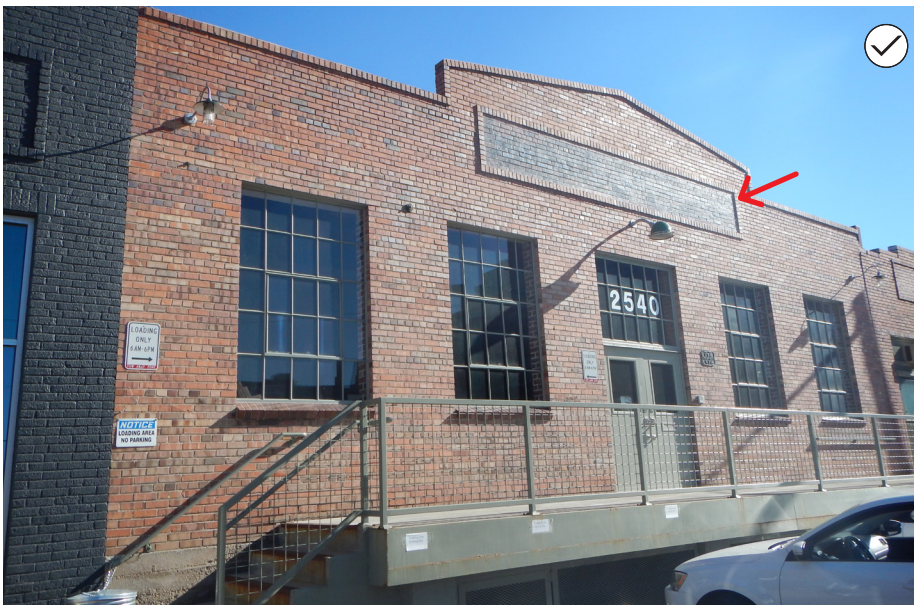
2. This building has an original sign band centered over the front door which would be a good signage location for a future user.
