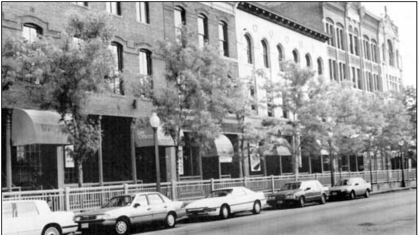
1600 block of Market Street across the street from the Market Street Transit Station. Leese 1991
