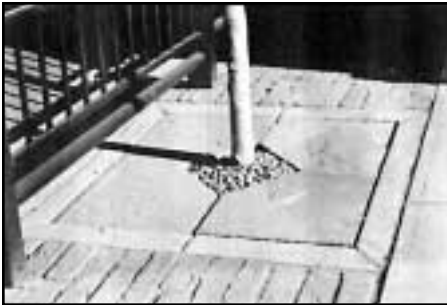
A flagstone tree well cover on 14th Street. MacIenman 1991
