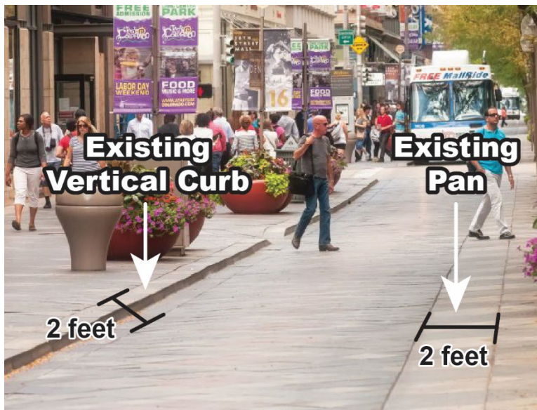
Figure 5-9. Existing Vertical Curb and Existing Pan on Median Block
