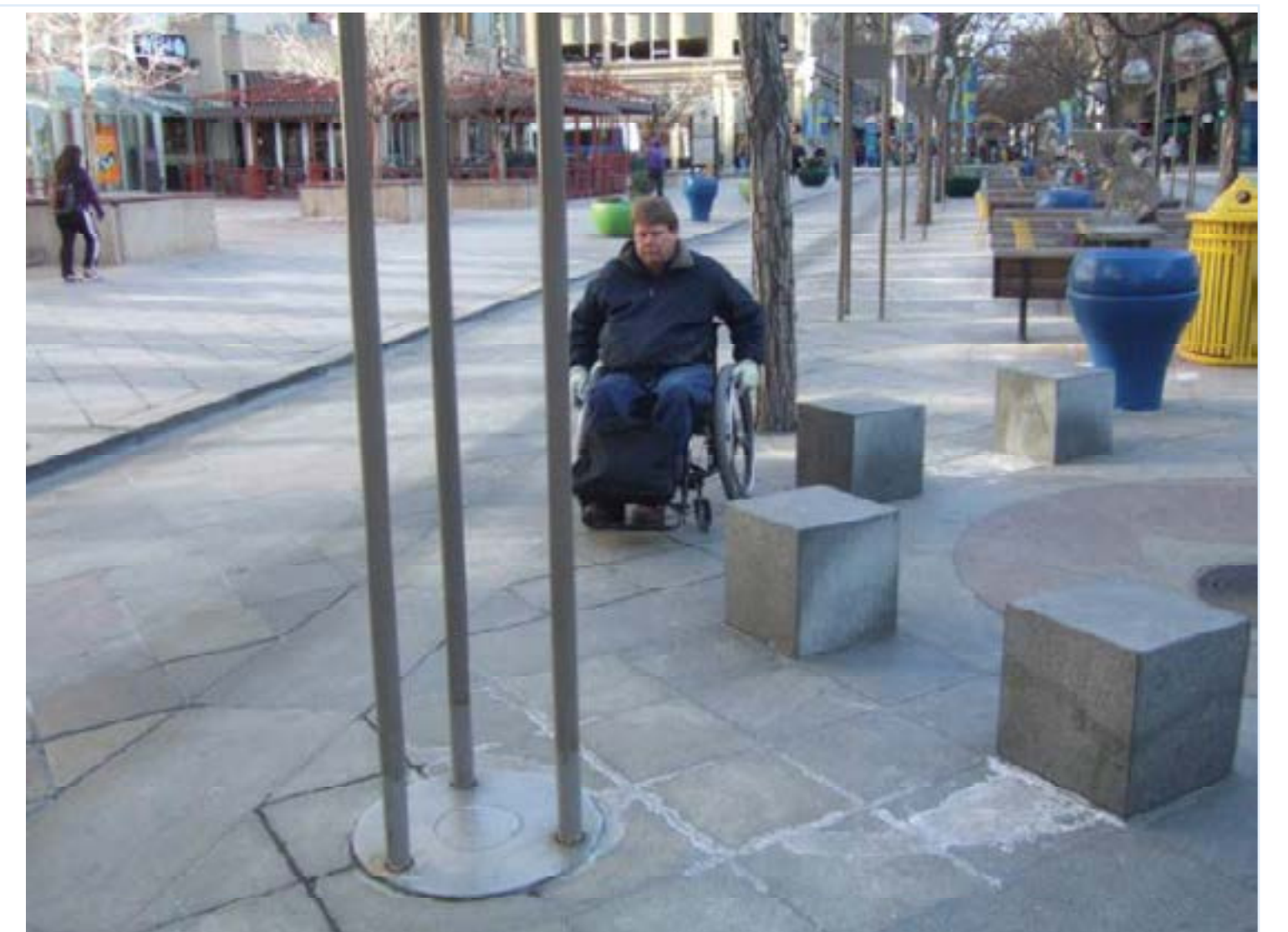
Less than 3' clear at median fountain
