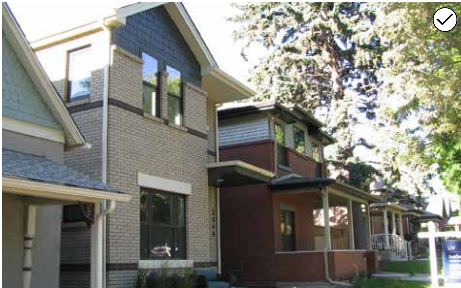
90. Standard brick in compatible color palette with shingle and lap siding accent materials.
