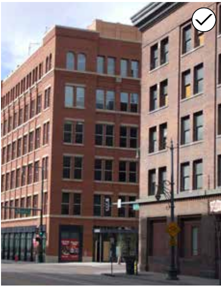
94. Incorporate windows, doors and other openings at a ratio similar to those found on nearby historic structures.
