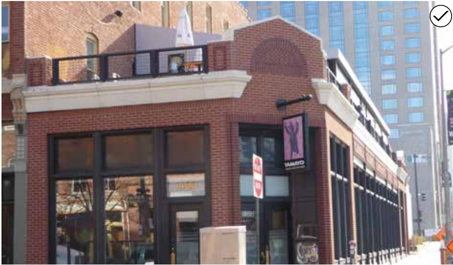
119. When locating a rooftop patio on a new building, minimize visual impacts on the streetscape.
