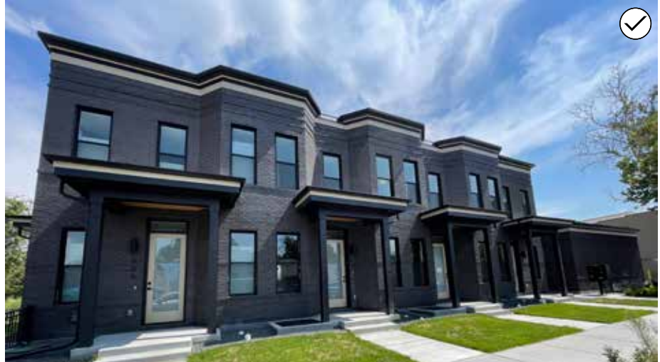
104. Use façade articulation techniques to help a new duplex, town house, or other small-scale residential building fit within the scale of the surrounding historic context.
