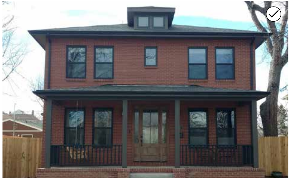
95. Incorporate windows, and doors at ratio similar to those found in the surrounding context.
