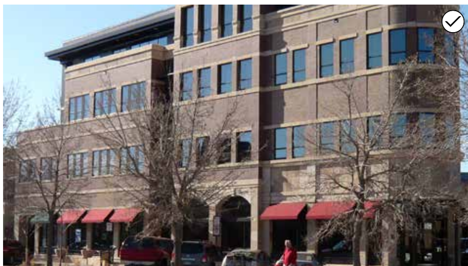
113. Use vertical and horizontal articulation design techniques to reduce the apparent scale of a larger building mass.
