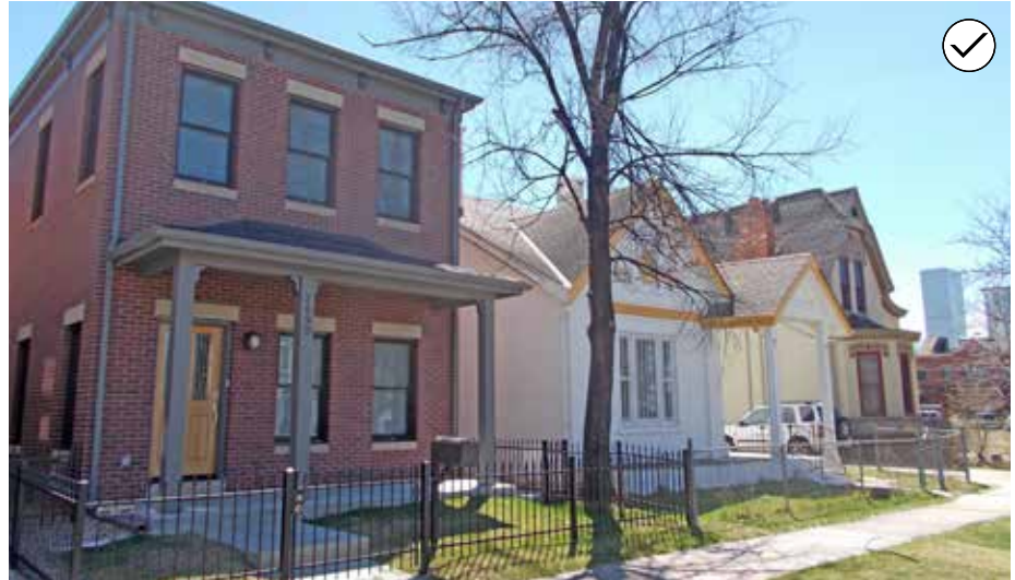
84. Where front yard setbacks are uniform, place a new structure in alignment with its neighbors.
