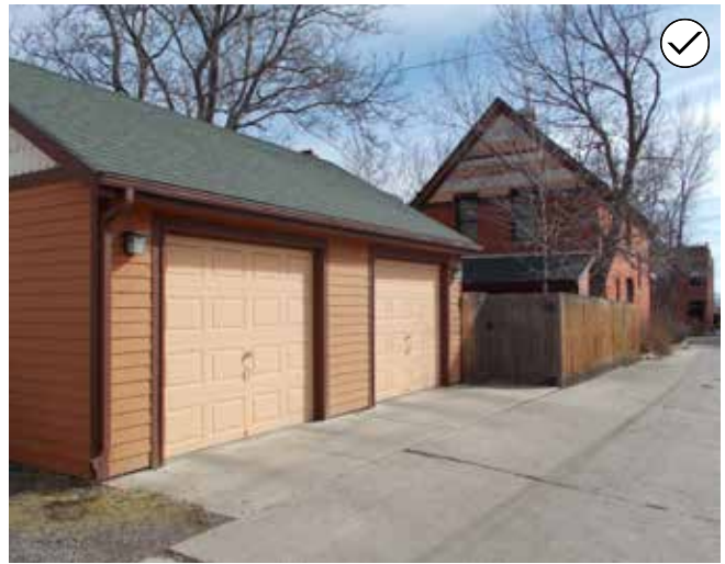
109. Design a new garage or secondary structure to be compatible with, and subordinate to, the primary structure and surrounding historic context.
