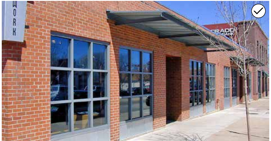
125. When introducing a new building into a historic district, it is also appropriate to consider incorporating sustainable design features that are typical of buildings in the surrounding historic context, such as canopies to provide shade.
