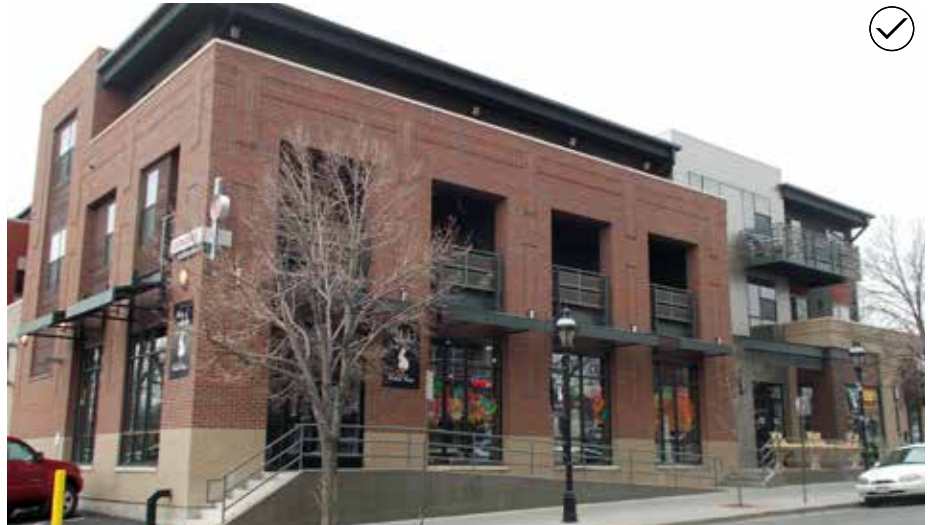
122. Divide the mass of a larger building into subordinate modules to reduce its perceived scale.
