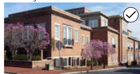
87. Use vertical and horizontal articulation techniques to reduce the apparent scale of a larger building mass.
