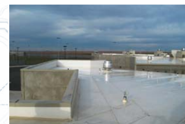
Light Reflecting Roofing over 100% of Roof Area.
