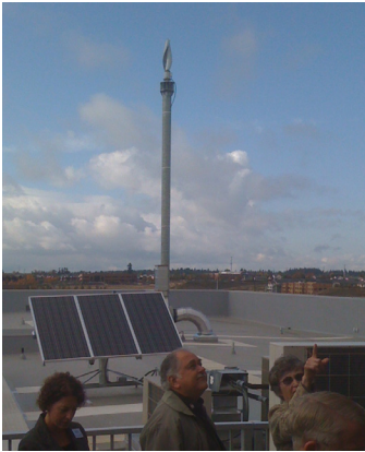
PV and Micro Wind turbines
