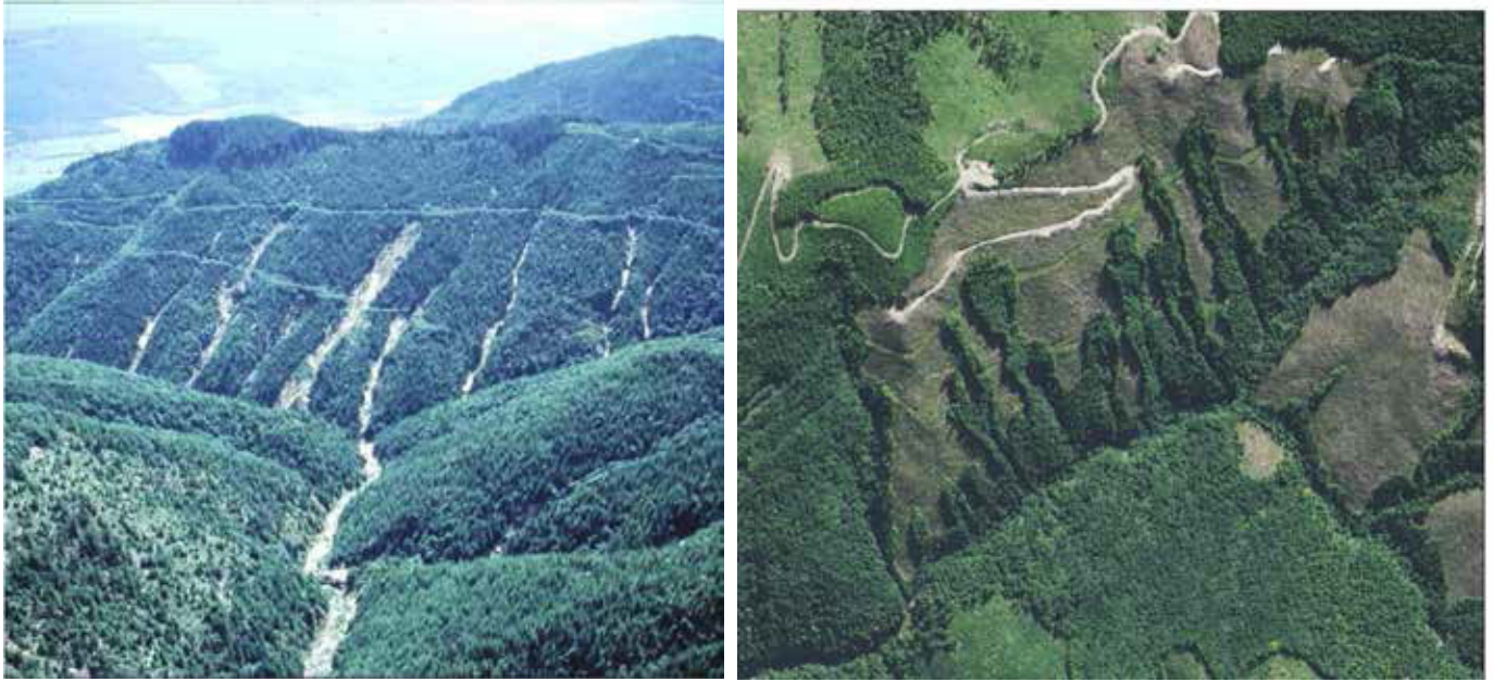
Figure 34. Left: Road-initiated debris flows in inner gorges unstable landforms, Sygitowicz Creek, Whatcom County (Photo: DNR, 1983). Right: Same hillslope 28 years later (2011 aerial photo).
