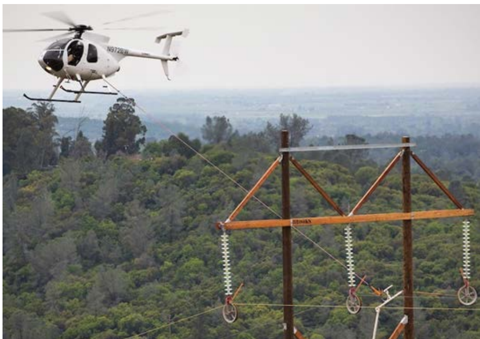
This H-frame transmission structure in California was built by Brooks Manufacturing. Photo/Brooks Manufacturing
