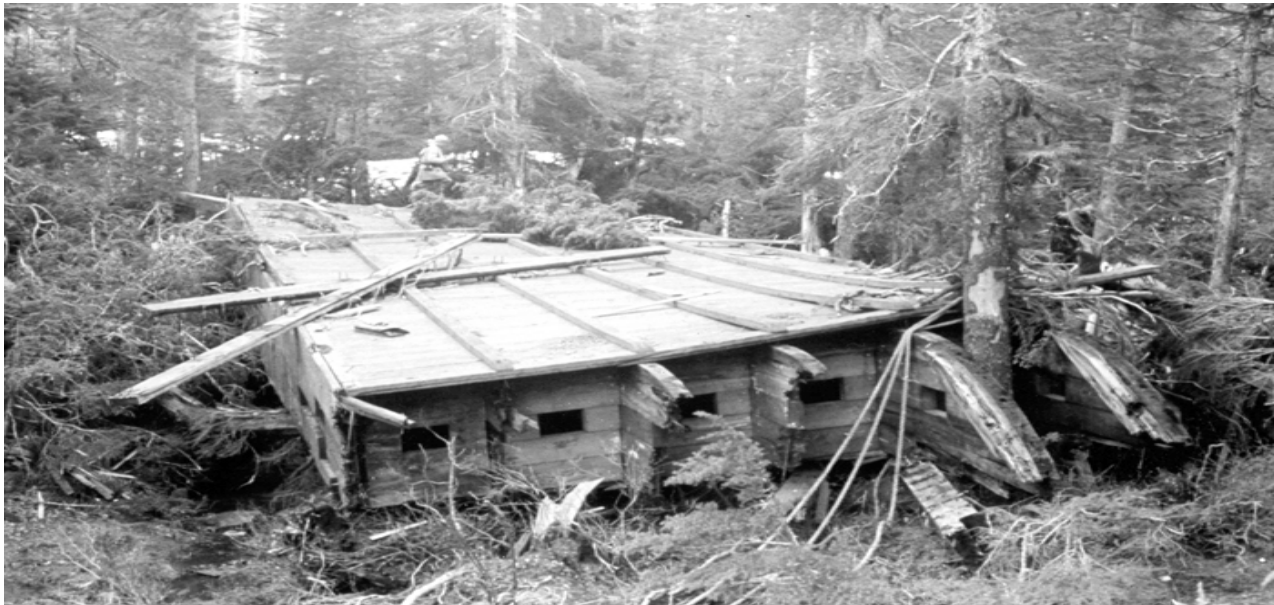
Alaska Earthquake March 27, 1964. Barge, 60 feet long and 25 feet wide, was broken loose from its mooring by a violent local wave in Port Nellie Juan, turned upside down, and deposited among the trees 200 feet from the shoreline about 30 feet above mean lower low water. Photo by G. Plafker, 1964. Figure 16, U.S. Geological Survey Professional Paper 542-G. Professional Paper-0542 Digital File:ake00003 From: http://137.227.241.37/cgi-bin/libcginw.cgi?SAME=1001Alaska+Earthquake+m%40Alaska+Earthquake+1964%40
