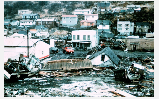
Tsunami damage at Kodiak, Alaska, following the 1964 Great Alaska Earthquake and Tsunamis (Credit: NOAA)
