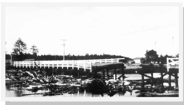
Figure 1: Bridge collapse after the tsunami debris came down the Copalis River (Credit: U.S. Army Corps of Engineers)
