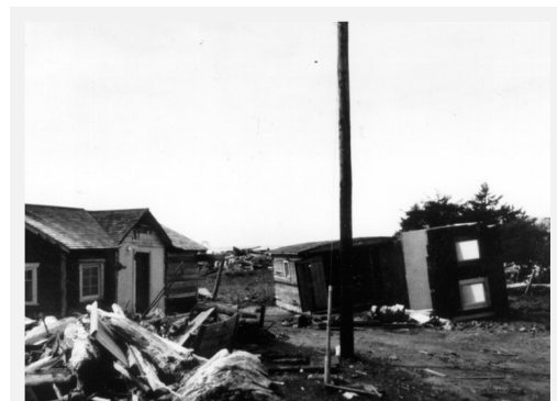
Figure 3: House torn apart from tsunami debris in Pacific Beach, Grays Harbor County (Credit: U.S. Army Corps of Engineers)
