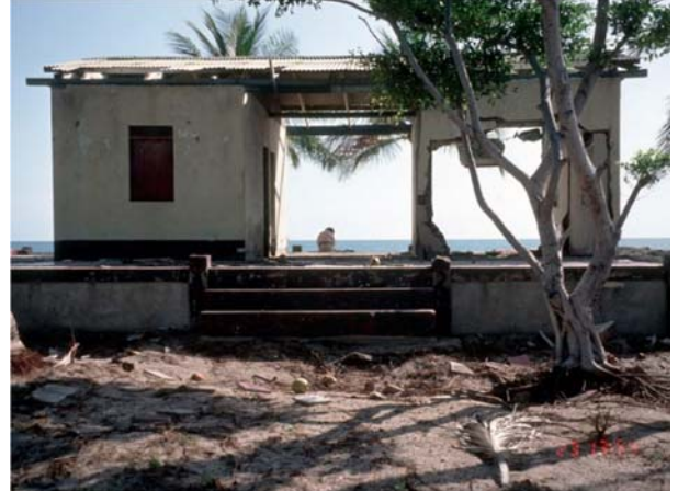
A photograph taken near the town of Popoyo, Nicaragua, during a post-tsunami survey following a M_w = 7.7 earthquake that struck Nicaragua's Pacific coast on 1 September 1992 local time. Here sedimentologist Jody Bourgeois, part of the first ever International Tsunami Survey Team (ITST), takes notes 3 weeks after the event at a house destroyed by the tsunami. Tsunami wave height reached almost 6 meters in this coastal town; most houses were washed away. Credit: Harry Yeh/NCEI
