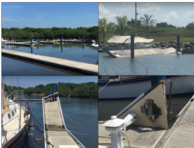
Figure 1: Video screen captures of dock damage in Marina Chiapas the day after the September 7, 2017, earthquake. According to the videographer, the amplitude of the tsunami in this area was several meters causing the floating docks to overtop the piles, and damage to the docks themselves (video link: https://www.youtube.com/watch?v=bBBVtIwLM9g ).
