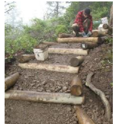
These box steps were built as part of a trail restoration project and will help minimize erosion by providing a stable and water-permeable hiking surface.
