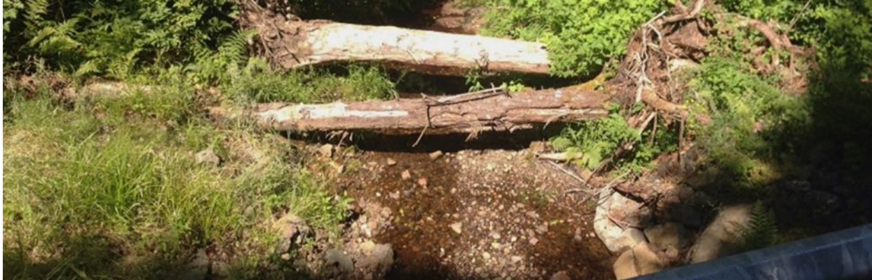
Figure 9: Large Down Woody Debris Left as Mitigation for a Road Crossing a Type 3 Stream. Photo courtesy of Zak Thomas.
