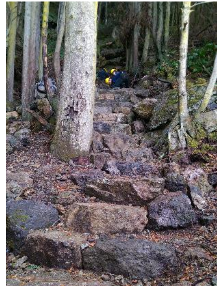
Figure 27: Installation of Rock Steps on Striped Peak Trail. Photo courtesy of Justin Zarzeczny.
