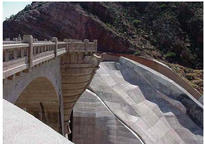
Coolidge Dam – San Carlos Irrigation Project
