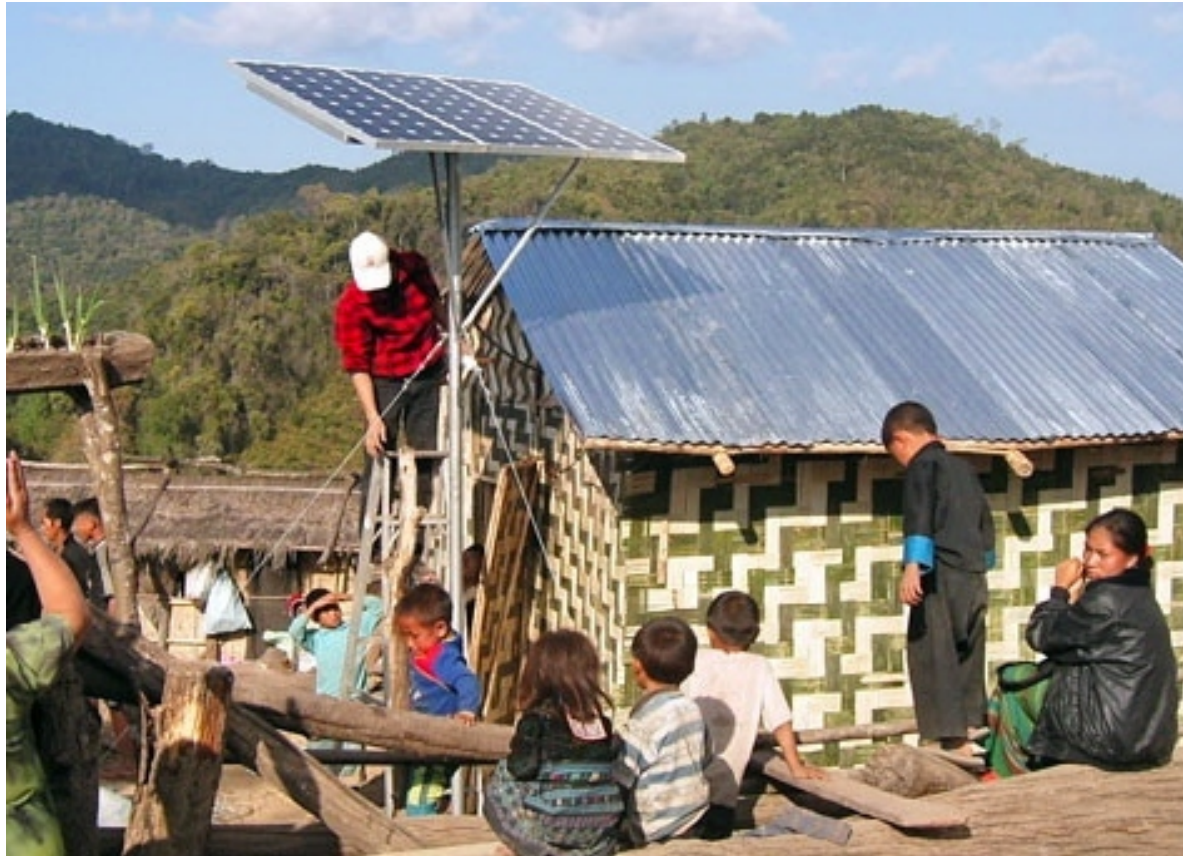
Upgrade and renovation
