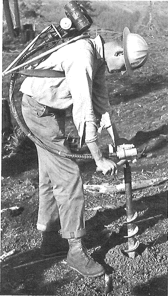
Figure 19. Auger-type machine boring a hole for planting.
