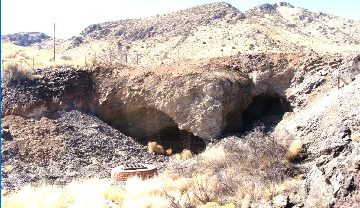
Lake Valley – Highwall Covered With Wire Mesh Fabric
