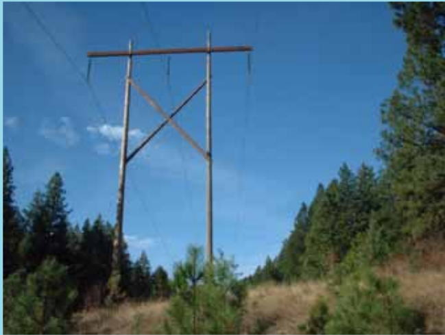
FIGURE 5: 115-kV line (3-phase)
