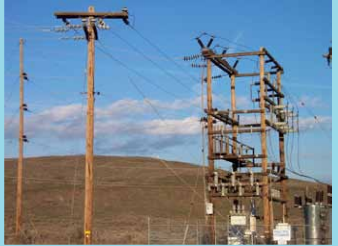
FIGURE 4: 69-kV to 34.5-kV (3-phase)
