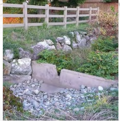
A roadside swale captures and retains runoff in Seattle, Washington. The city saves money with LID by avoiding costly stormwater infrastructure and reducing paving costs.
