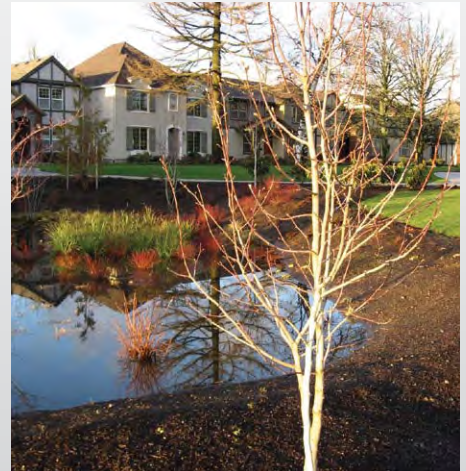
This bioretention pond in Wilsonville, Oregon collects runoff from the rooftops, sidewalks and yards. The pond offers valuable aesthetic and wildlife habitat benefits while also reducing stormwater control costs.
