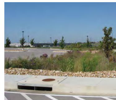
Street drainage flows into this roadside bioswale in Lenexa, Kansas. The city found that on-site detention with LID practices cost 25 percent less than traditional stormwater management retrofits.
