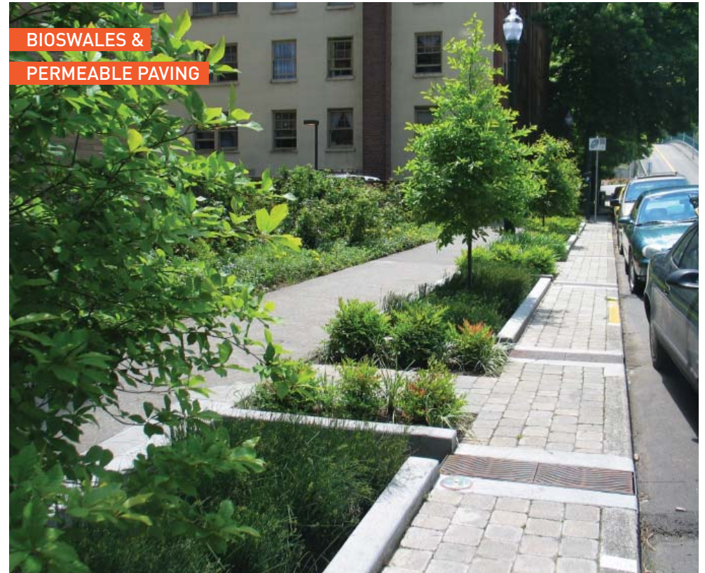
FIGURE 45 Green streets of Portland, Oregon. The use of rain gardens along city streets acts as a buffer between vehicular and pedestrian right of way. Bioswales and permeable paving store storm water runoff and clean the water before entering the storm drainage system.
