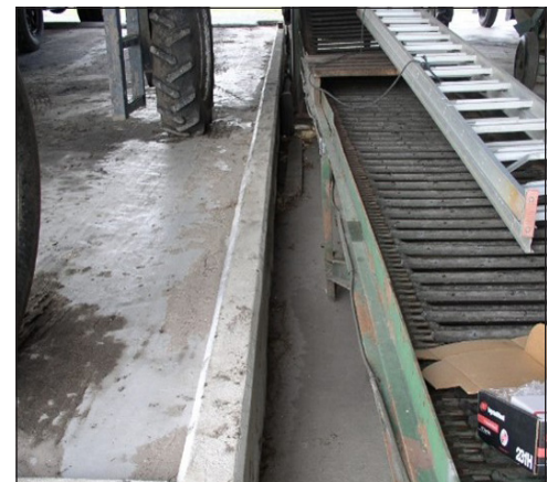
Containment of spillage part of the Ag. Chemical Facilities.
