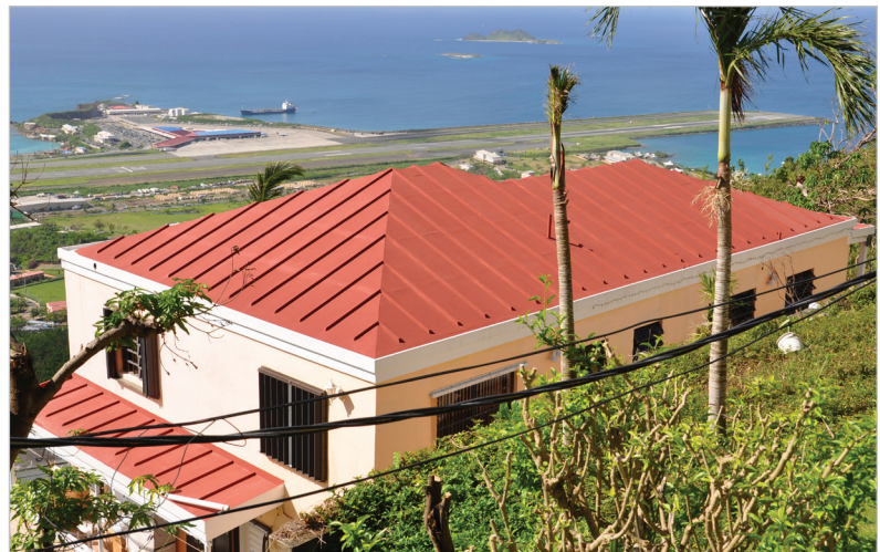
Figure 3-5: A liquid-applied membrane over plywood with wood battens roof system.
