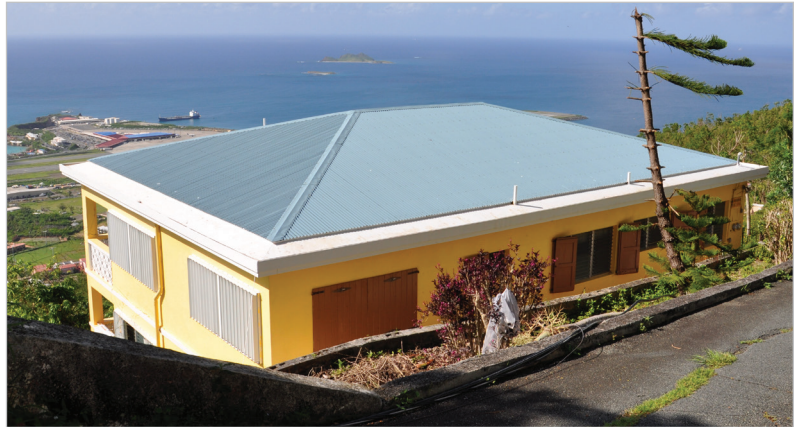
Figure 3-4: A corrugated metal panel roof with integral gutter.
