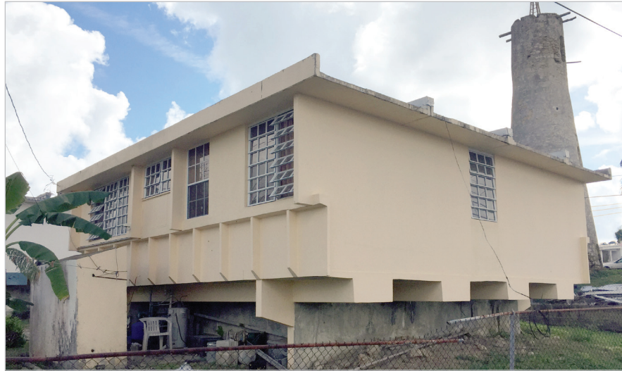
Figure 3-6: Typical Sion Farm home constructed of pre-cast concrete wall and roof panels.
