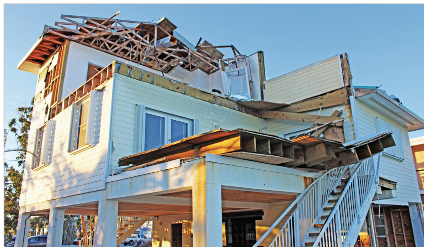
Figure 3-8: House with wind damage.
