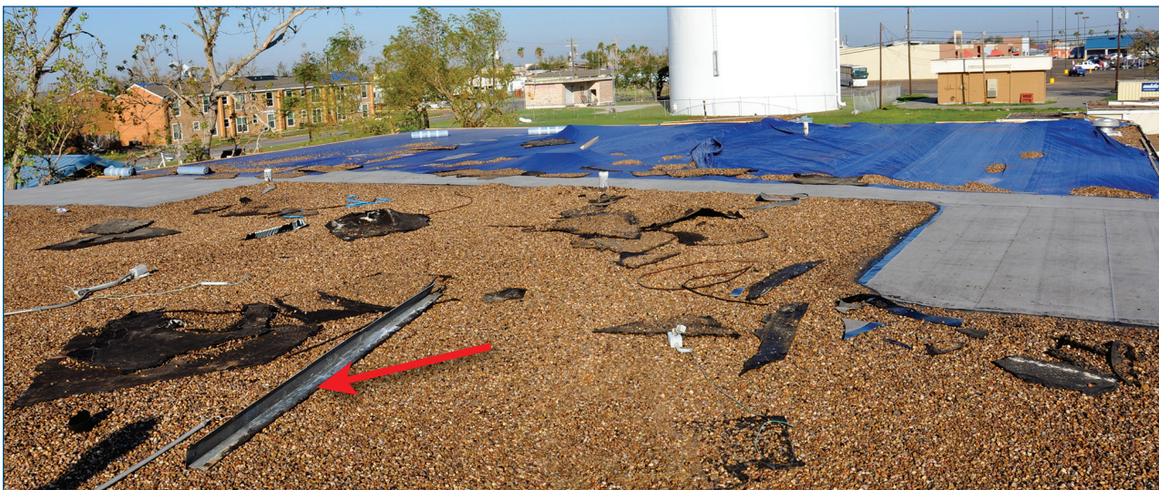
Figure 3-10: View of emergency repairs
