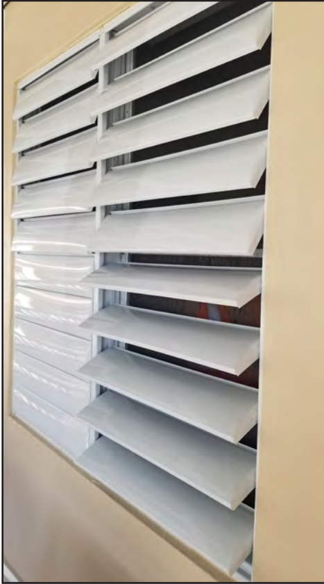
Figure 3-40: Close-up of jalousie windows with metal louvers on a residential building.
