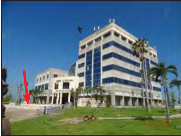
Figure 5-60: Toa Baja Municipal Building showing relief from surrounding terrain by use of elevation on fill. Stairs lead to the building's elevated pad (red arrow).
