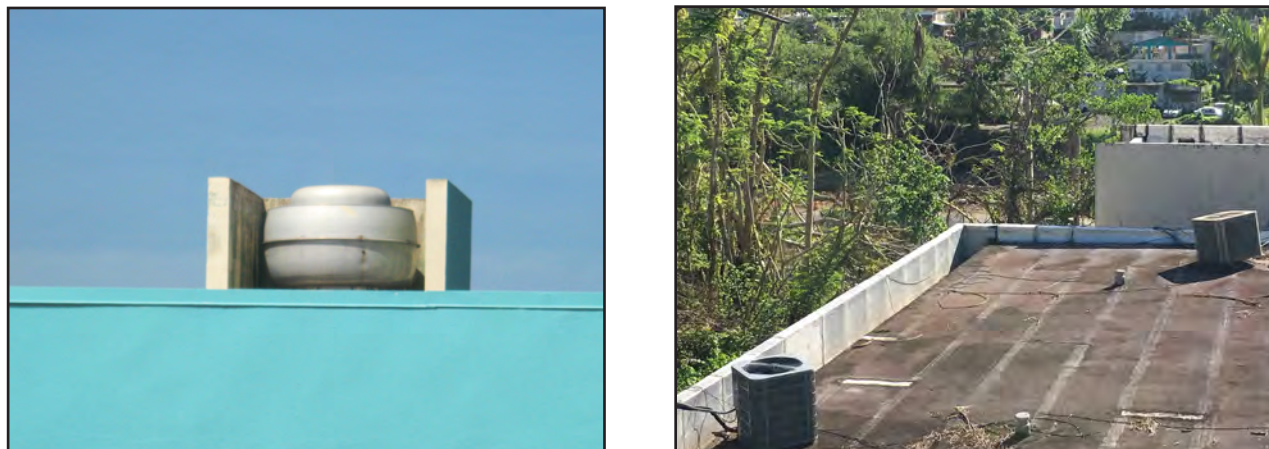
Figure 4-28: Left, Jose Robles Otero Elementary School had concrete walls that may have shielded rooftop equipment from wind. Right, small rooftop equipment at Eduardo Garcia Carrillo High School in Canóvanas was not properly secured and was displaced by wind forces from Maria.
