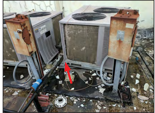
Figure 5-82: View of rooftop mechanical equipment displaced and damaged by the hurricane winds. Left, the access panels were blown off (yellow circle). Right, the units were moved off their mounting pedestals (red arrow).
