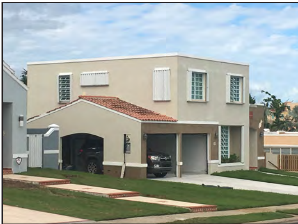
Figure 3-35: Concrete residences in, left, Palmas del Mar; right, Loíza, that performed well with no structural damage.
