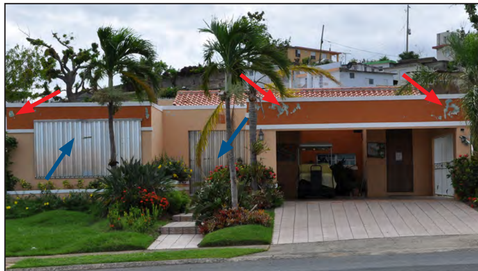
Figure 3-47: Residential building with metal panel shutters over windows and exterior doors (blue arrows). Damage is visible on exterior finish (red arrows).
