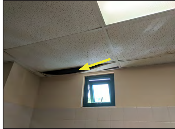
Figure 5-76: Membrane roof covering at Culebra City Hall punctured (red arrow) during hurricane winds led to water intrusion in building that damaged acoustical ceilings (yellow arrow) and drywall.
