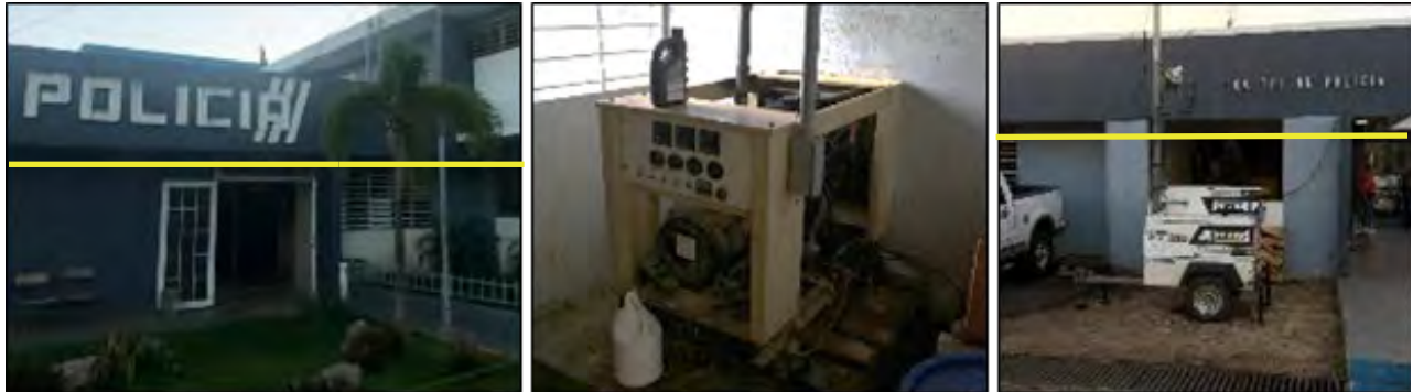
Figure 5-44: Corozal Police Station, left, overview; center, damaged backup generator; right, portable generator used after Hurricane Maria. Yellow line indicates high water mark.
