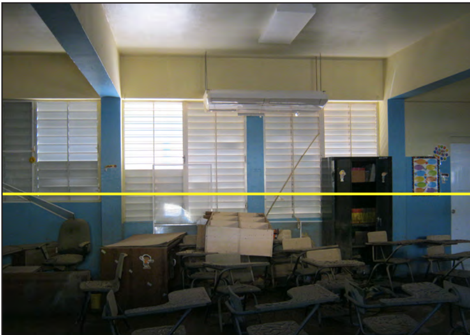
Figure 4-7: Classroom at Luis M. Santiago School with high-water line indicated (yellow line).
