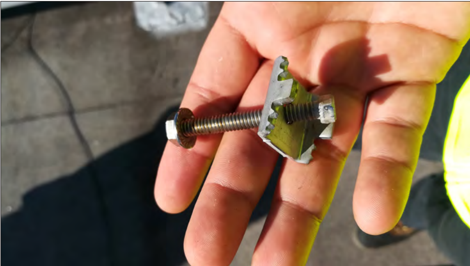
Figure 6-31: Side view of clamp used to attach adjacent PV panels to frame.
