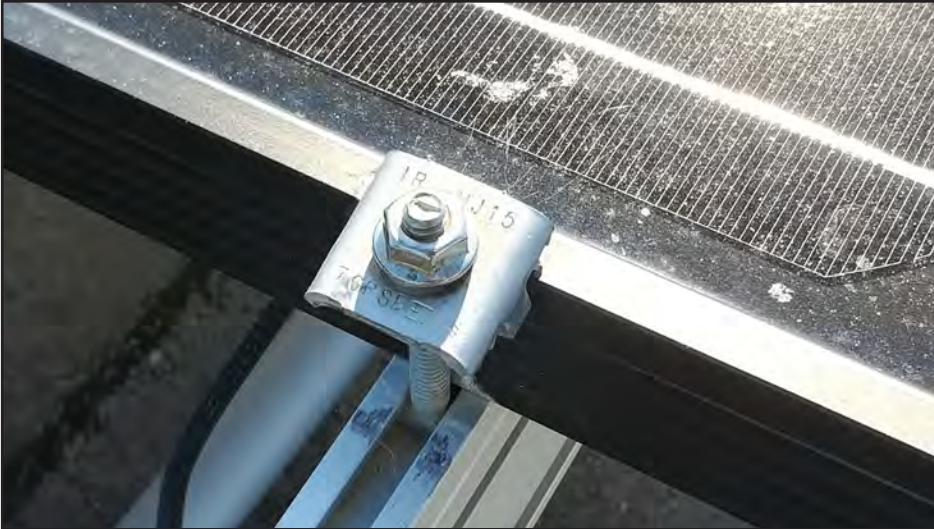
Figure 6-30: Clamp used to attach adjacent PV panels to frame.
