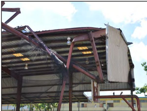
Figure 4-16: Left, the end bay of this MBS athletic facility failed when it could not resist wind pressures during Hurricane Maria. Corroded structural members, right, likely contributed to the failure. In this column, a hole had formed in the web (red arrow).
