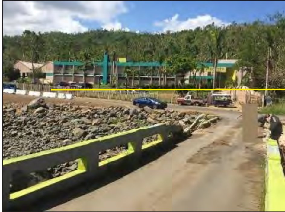
Figure 4-5: Floodwaters from the stream under this bridge rose to the edge of the mapped Zone AE (yellow line) in the parking lot immediately adjacent to the school. The floodwaters did not enter the school.
