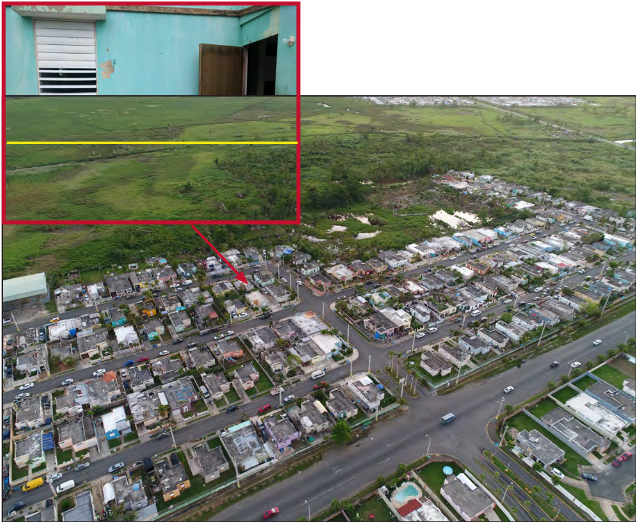
Figure 3-73: Aerial image of Campanilla NSHP community, Toa Baja. The community was elevated on fill, resulting in isolation of properties during Hurricane Maria due to flooding of surrounding areas. Homes on the southern portion of the community experienced shallow flooding. Zone AE. Inset, NSHP home in Campanilla showing approximate inundation depth (yellow line).
