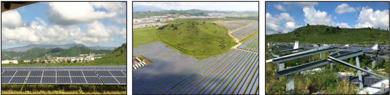
Figure 6-2: High wind damage to ground-mounted photovoltaic (PV) systems in the Reden Solar Array, Humacao, showing panels in Phase 1, left; hill separating the two phases, center; and Phase 2, right.
