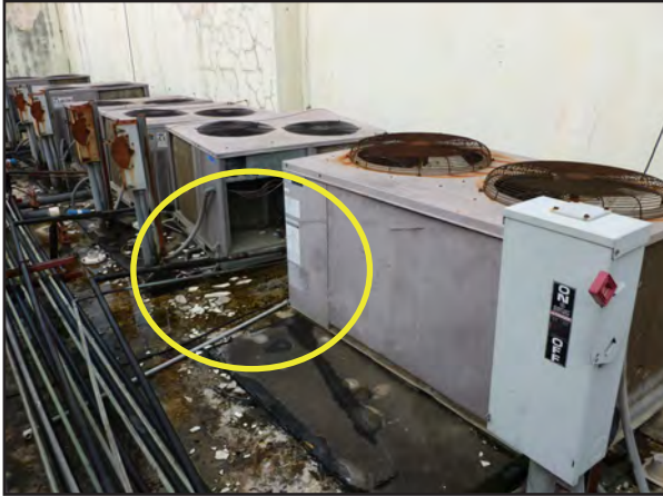
Figure 5-82: View of rooftop mechanical equipment displaced and damaged by the hurricane winds. Left, the access panels were blown off (yellow circle). Right, the units were moved off their mounting pedestals (red arrow).
