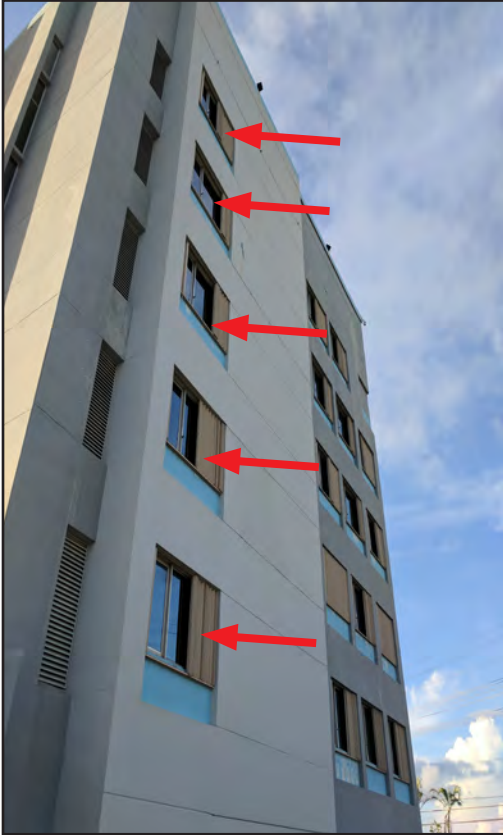
Figure 5-71: Vega Alta Municipal Building had shutters on only the east side windows (red arrows). No shutters or opening protection is present on windows on this side of the building.
