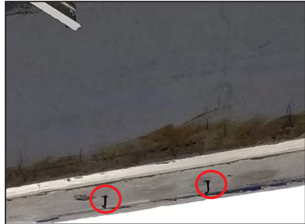
Figure 5-68: The screws that held the window frame in place bent and pulled through the window frame at the PRDOJ building. The anchors (red circles), were too small and too few in number.
