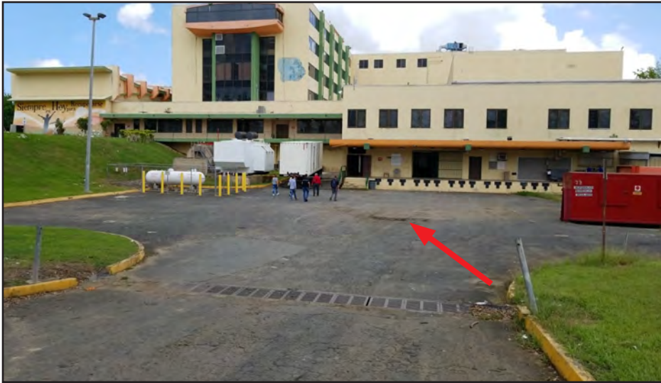
Figure 5-6: The loading dock area at Dr. Ramon Ruiz Arnau University Hospital flooded when the area drains (red arrow) were overwhelmed by surface runoff.
