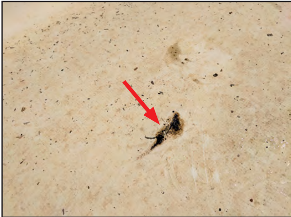
Figure 5-76: Membrane roof covering at Culebra City Hall punctured (red arrow) during hurricane winds led to water intrusion in building that damaged acoustical ceilings (yellow arrow) and drywall.
