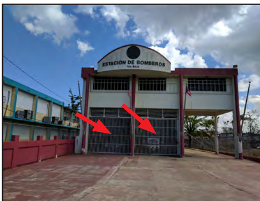
Figure 5-48: Toa Baja Fire Station. Left, security grilles (red arrows) protected equipment from wind-borne debris. Right, metal shutters (blue arrows) protected the building from wind-borne debris.
