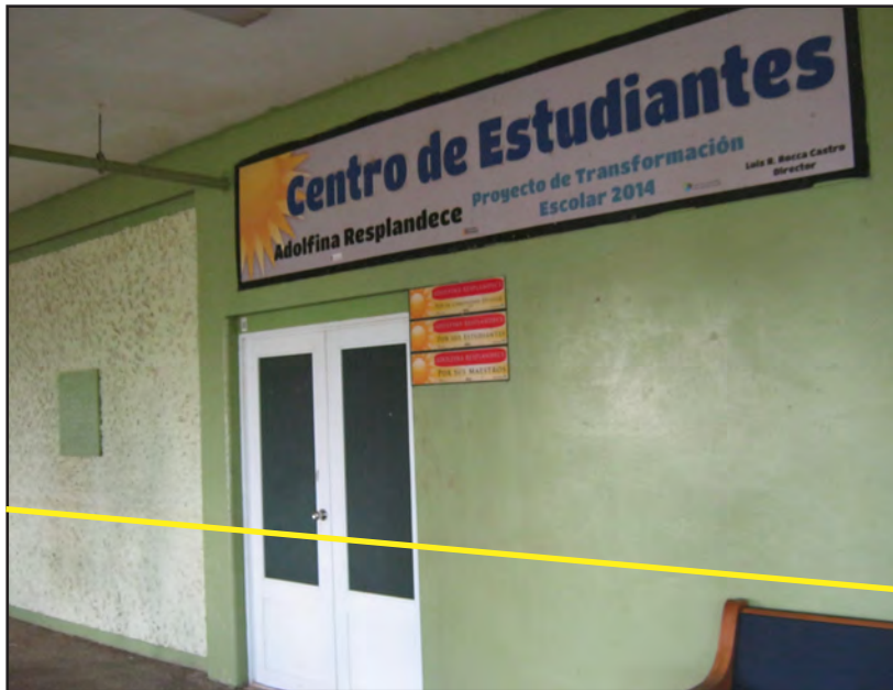
Figure 4-9: Toa Baja High School building student center area underneath the elevated building that flooded during Maria. The school received 2.5- 3 feet of flooding (yellow line).
