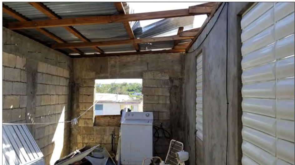
Figure 3-50: Metal roof covering with no structural decking.
