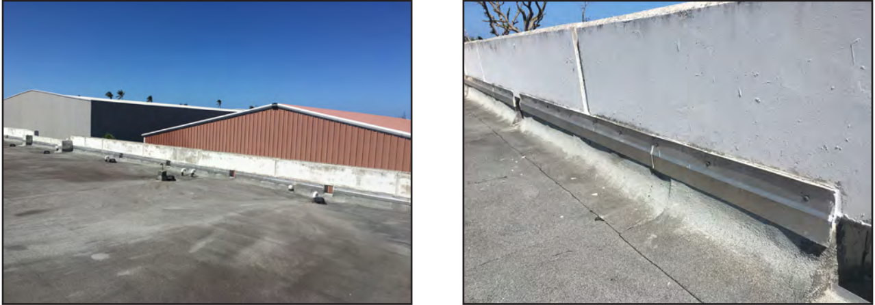
Figure 4-21: Modified bitumen roof covering at a high school in Loíza.
