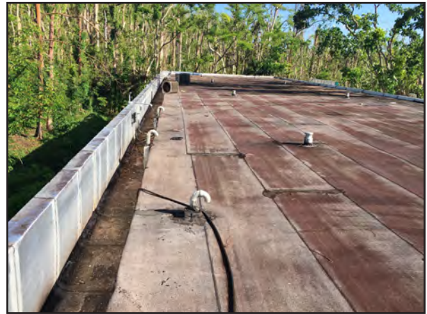
Figure 4-12: Eduardo Garcia Carrillo High School, left, did not experience structural failures to reinforced concrete classroom buildings. Damage at these buildings was due to water intrusion from the roof, right, and through windows.
