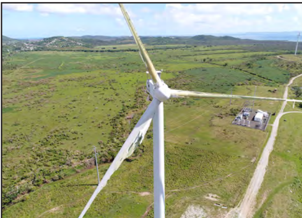
Figure 6-42: Wind turbines damaged by the hurricanes in Naguabo, along the northeastern coastline of Puerto Rico.
