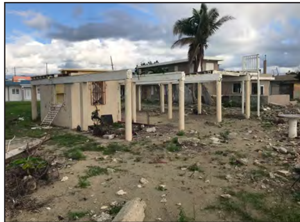
Figure 3-8: Left, concrete house in Fajardo subject to 1.5-foot (0.5-meter) wave heights. Current FIRM and Advisory Data: VE Zone. Right, elevated beachfront house in Punta Santiago, Humacao subjected to wave heights greater than 1.5 feet (0.5 meters). Current FIRM: AE Zone. Advisory Data: CAZ.
