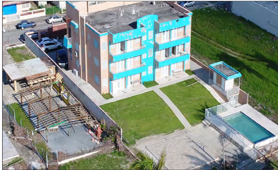
Figure 3-3: Apartment building in Punta Santiago, Humacao, elevated on fill. Adjacent buildings experienced significant damage from coastal storm surge. Effective FIRM: Zone AE. Advisory Data: CAZ.
