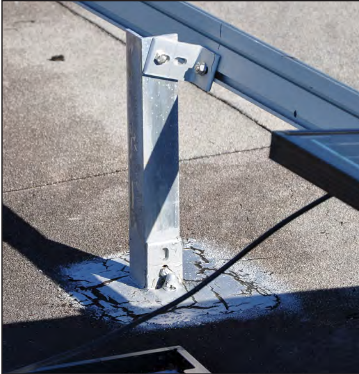
Figure 6-32: Close-up view of the anchoring connection to the roof concrete slab.
