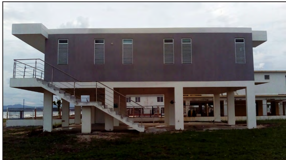
Figure 3-39: Elevated concrete residential building with glass jalousie windows.
