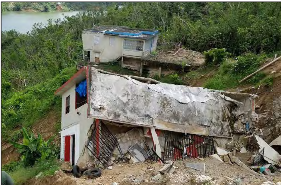
Figure 3-66: House that failed due to landslide in Utuado. Source: NWS (2017)
