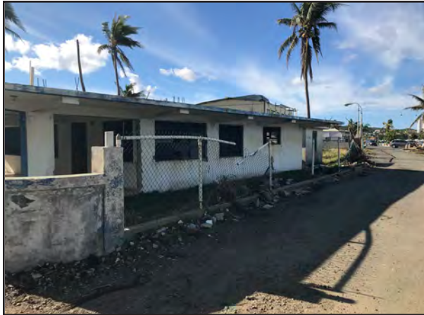
Figure 3-8: Left, concrete house in Fajardo subject to 1.5-foot (0.5-meter) wave heights. Current FIRM and Advisory Data: VE Zone. Right, elevated beachfront house in Punta Santiago, Humacao subjected to wave heights greater than 1.5 feet (0.5 meters). Current FIRM: AE Zone. Advisory Data: CAZ.
