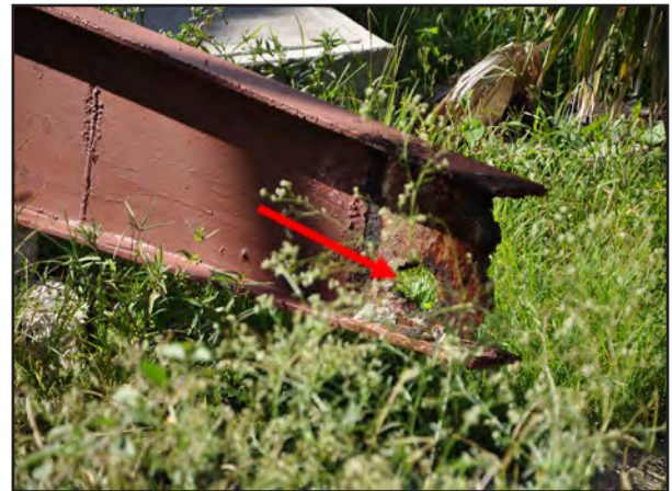
Figure 4-16: Left, the end bay of this MBS athletic facility failed when it could not resist wind pressures during Hurricane Maria. Corroded structural members, right, likely contributed to the failure. In this column, a hole had formed in the web (red arrow).
