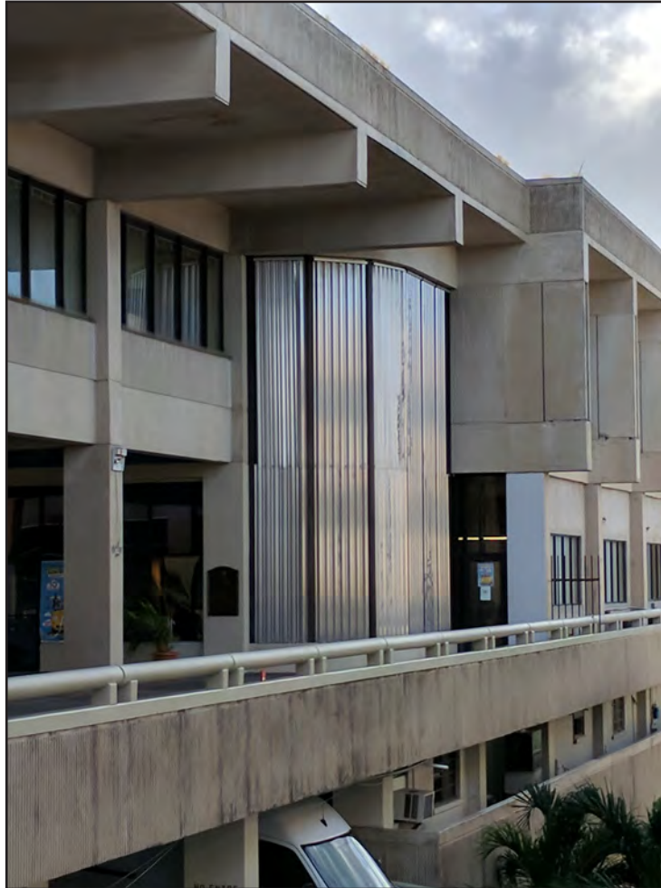
Figure 5-73: Metal shutters protected some upper-story glazed windows at Bayamón Municipal Building.
