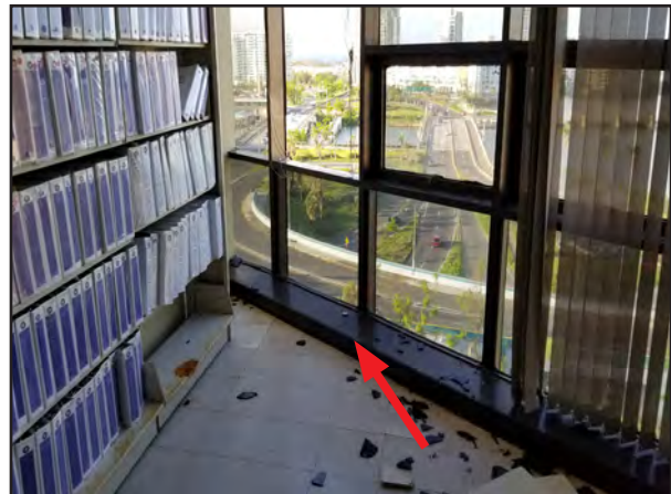
Figure 5-68: The screws that held the window frame in place bent and pulled through the window frame at the PRDOJ building. The anchors (red circles), were too small and too few in number.
