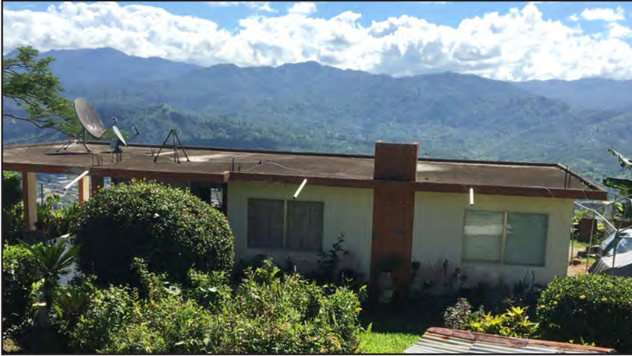
Figure 3-69: Hillside residence in Utuado that was sited away from the edge of the slope and designed to resist potential flood and wind forces.
