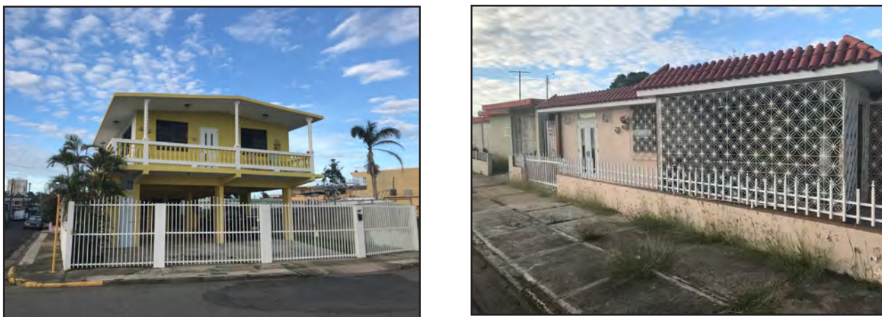
Figure 3-2: Elevated house (left) and non-elevated house (right) in northern Mayaguez, Zone AE.
