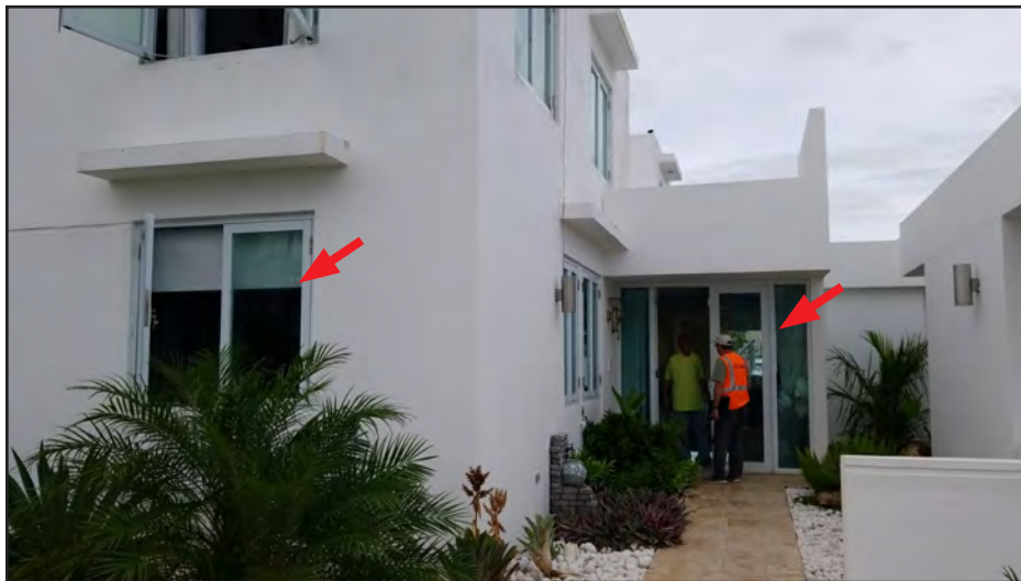
Figure 3-43: Concrete single-family home with impact-resistant glazing covering windows and doors (red arrows).
