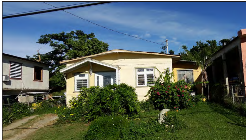
Figure 3-29: Example of a wood-framed home in Vieques that performed well during Hurricane Maria.
