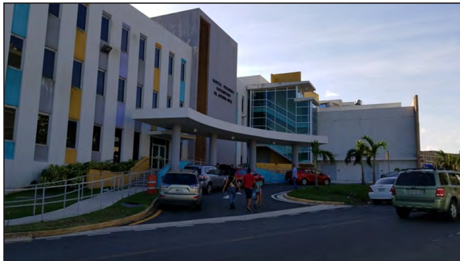
Figure 5-8: View of the front entrance of the San Juan University Pediatric Hospital.
