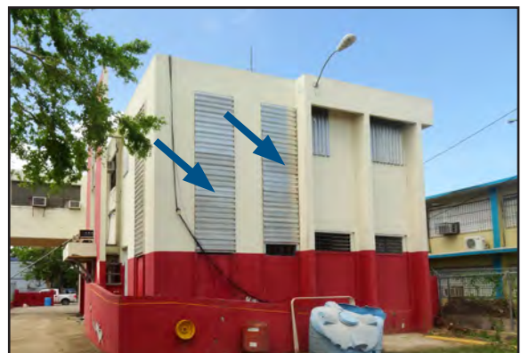
Figure 5-48: Toa Baja Fire Station. Left, security grilles (red arrows) protected equipment from wind-borne debris. Right, metal shutters (blue arrows) protected the building from wind-borne debris.
