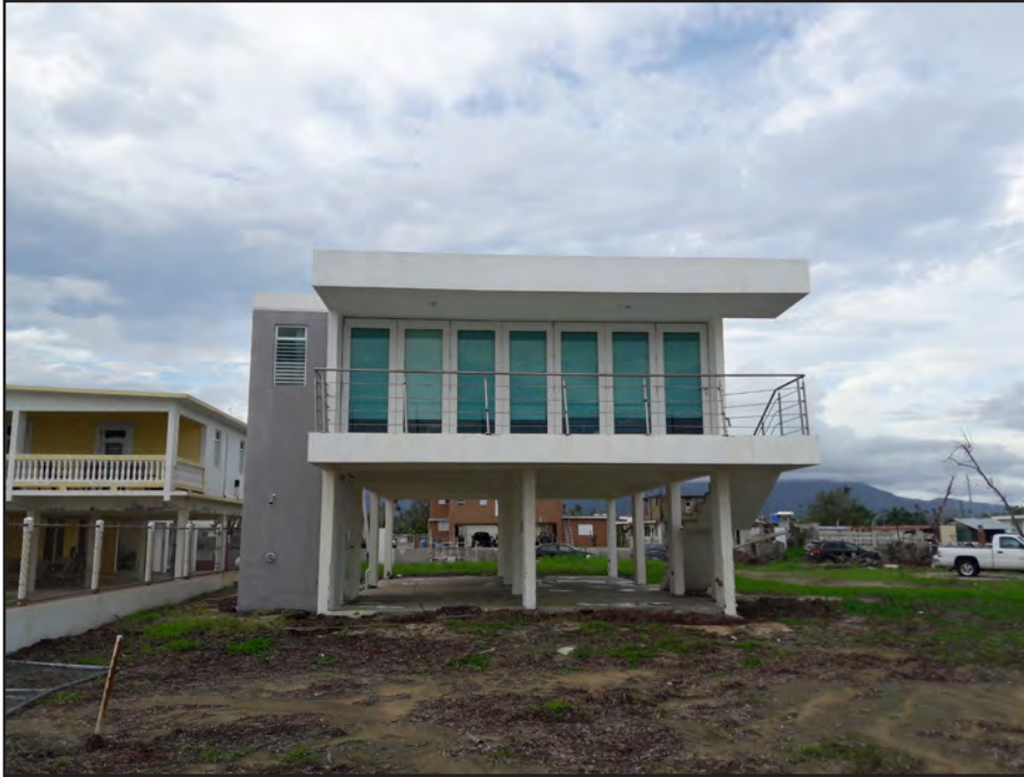
Figure 3-1: Elevated concrete house in Punta Santiago that performed well.
