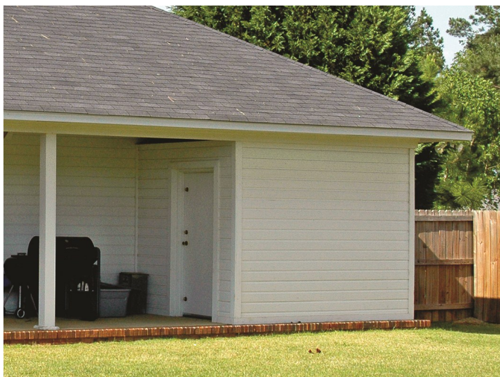
An above-ground safe room constructed as an addition to a slab-on-grade home in a way that matches the aesthetics of the home (Tuscaloosa, AL).
