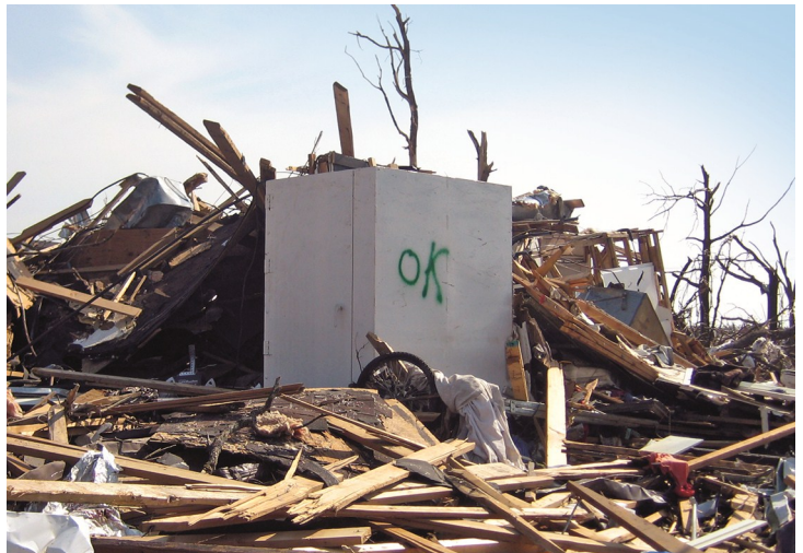
Above-ground residential safe room that was in the garage of a home hit by an EF5 tornado (Joplin, MO).
